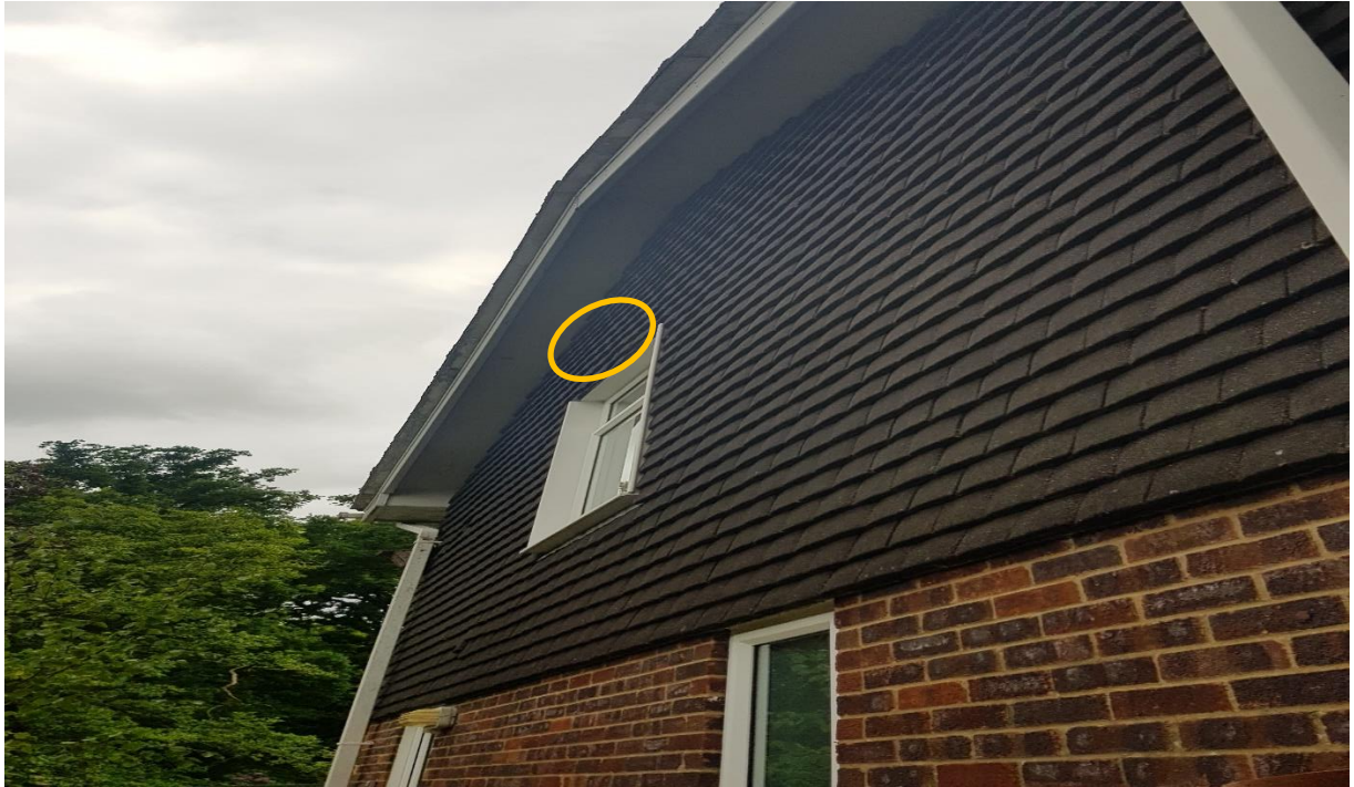
Figure 2: Showing the area the bats re-entered on the southern elevation
