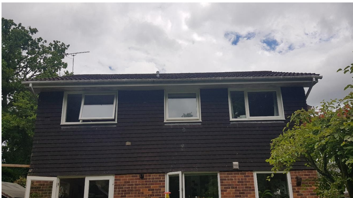
Picture 2: Showing the western (rear) elevation.
