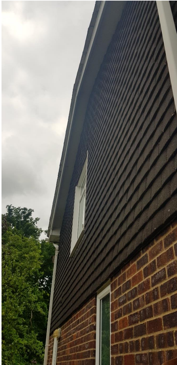
Picture 4: Showing the hanging tiles on the southern elevation
