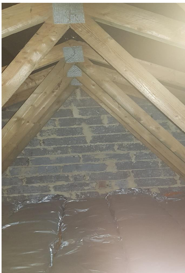
Picture 5: Showing the internal roof space
