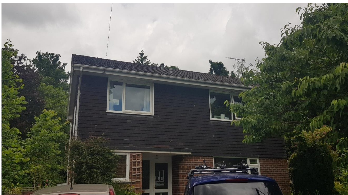
Picture 1: Showing the eastern (front)elevation
