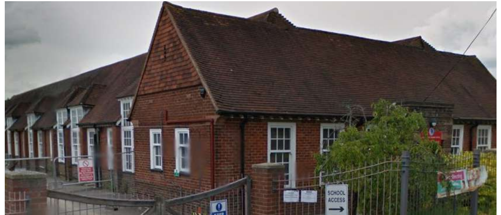
Crescent Primary School - brick walls, steep pitched tiled roofs.
