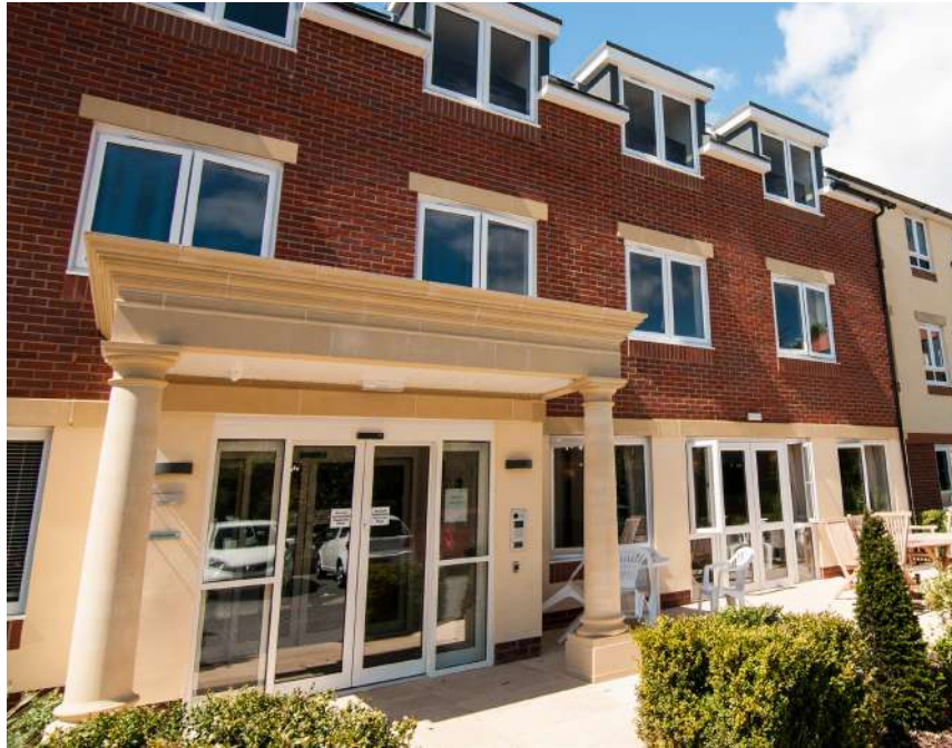
Secure Main Entrance from Parking
