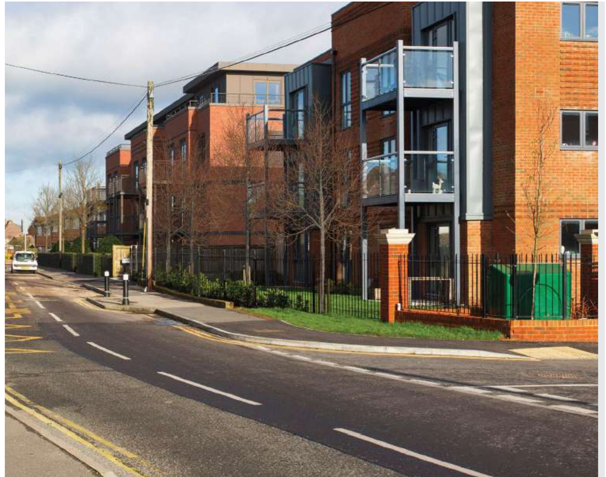
Verified View 2 - looking north along Toynbee Road
