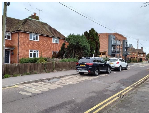
Photograph 6: Toynbee Road On-Street Parking and Double-Yellow Lines
