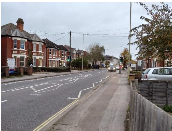
Photograph 13: Signalised Crossing along Leigh Road
