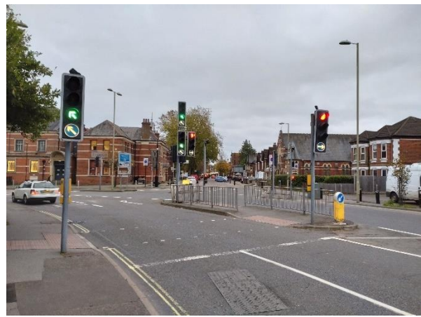
Photograph 14: Signalised Crossing at the Leigh Road/Romsey Road Junction
