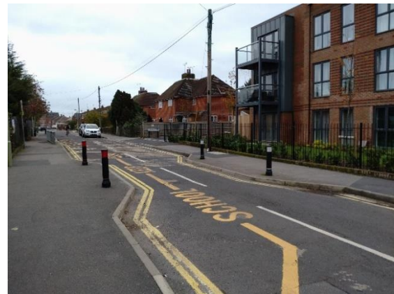
Photograph 4: Traffic Calming Measures along Toynbee Road
