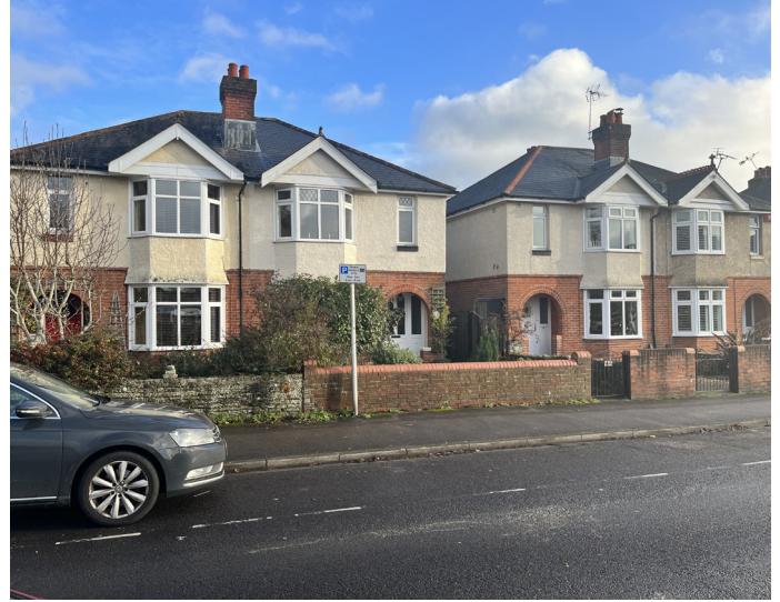
Red brick to ground floor with contrasting coloured render to first floor
