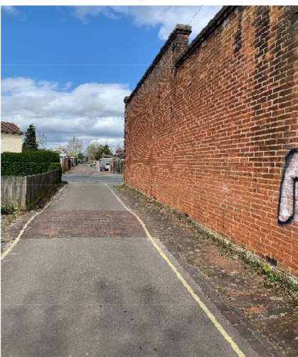
Image 5 – West Service Road looking north
