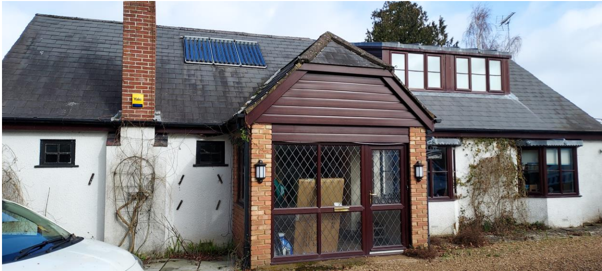
Photo 1: The main dwelling, southern aspect
