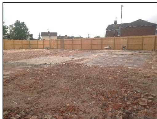
Figure 2: Hardstanding where demolished buildings once stood
