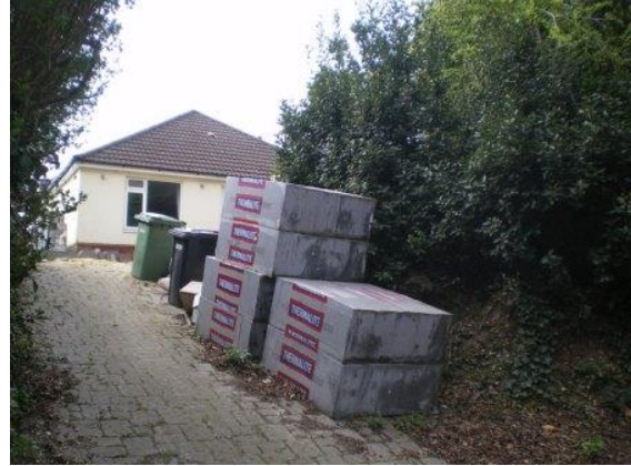
Photo 2. Front of Ramcrest viewed from Lowford Hill, facing south. (Taken 08/04/21)
