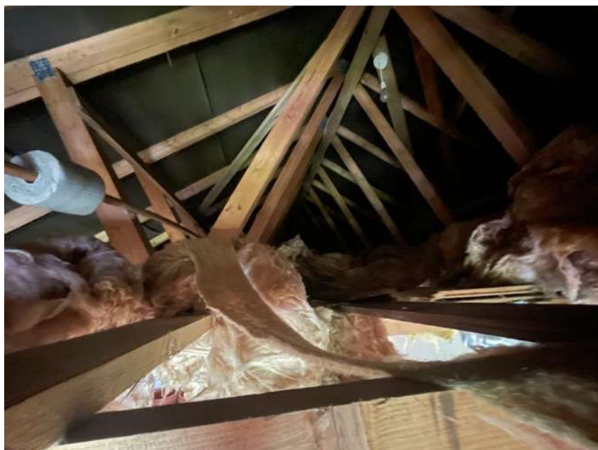
Figure 2. Photo of internal loft space showing intact underlining
