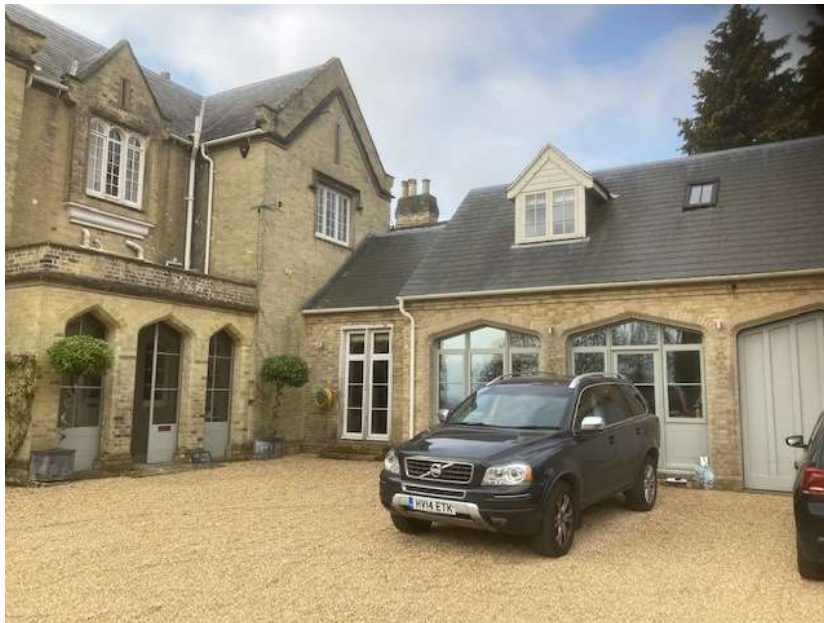
Fig.5 – Photograph showing the 'link' between the garage extension and the main house.
