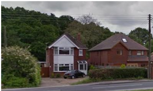
Image 3: Appeal property and frontage prior to renovation
