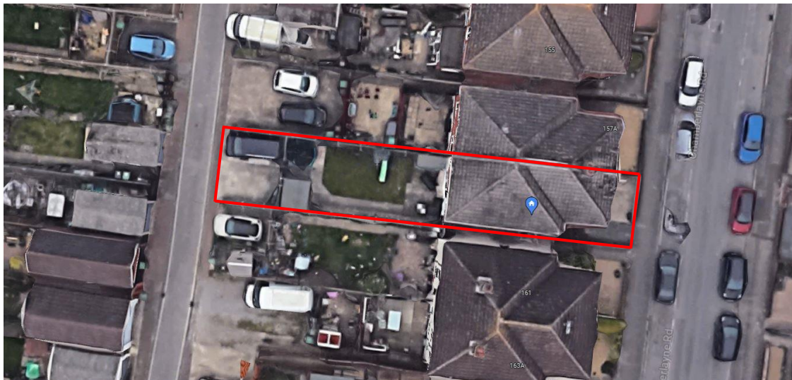
Site location aerial, back boundary service road.
