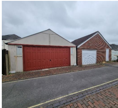
High pitched roofs abutting service Rd.
