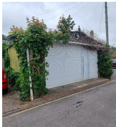
Garage abutting service Rd.
