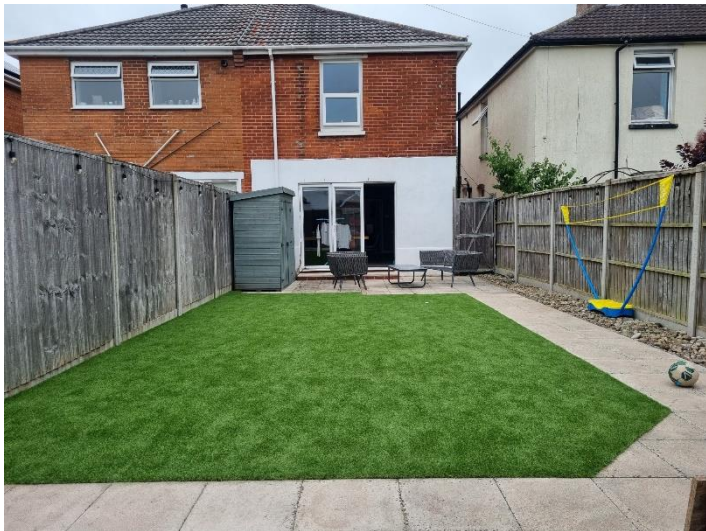
Rear elevation of existing dwelling facing West.
