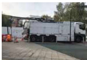
HIGH PRESSURE JETTING
