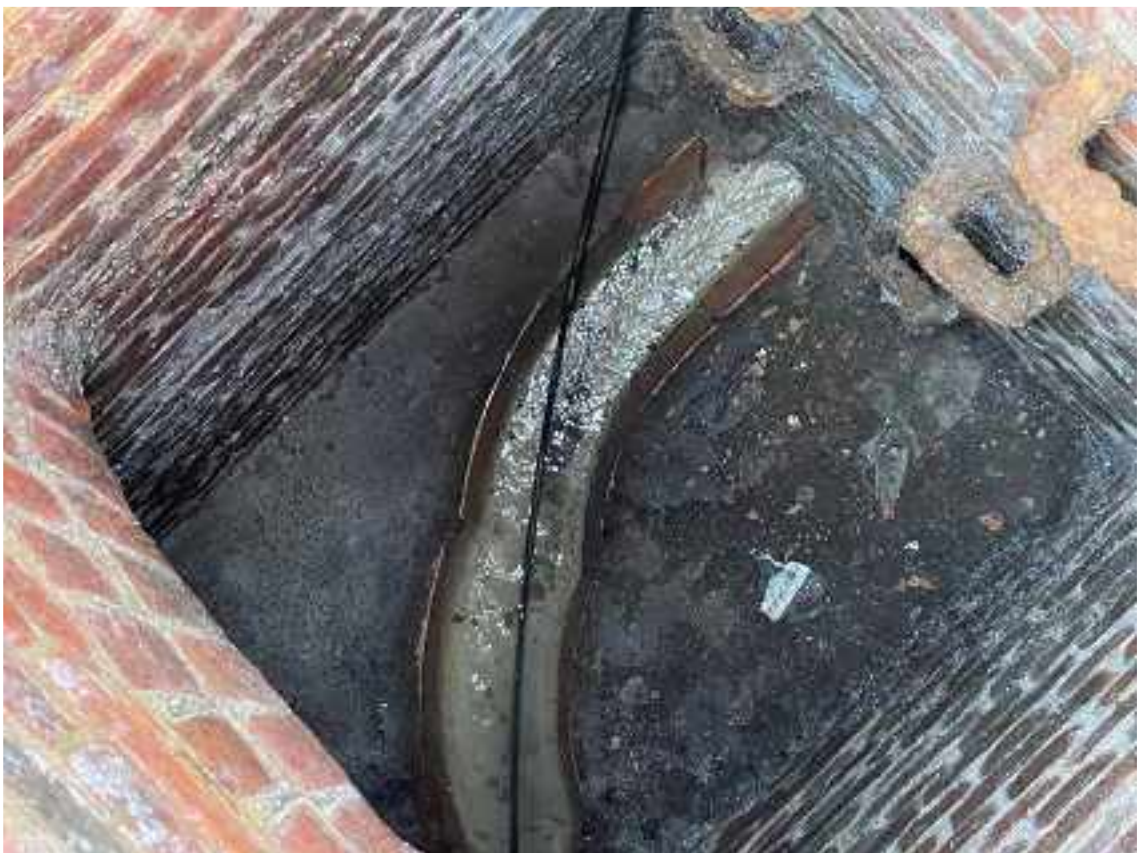
MH 2201 (CLOSE UP)
