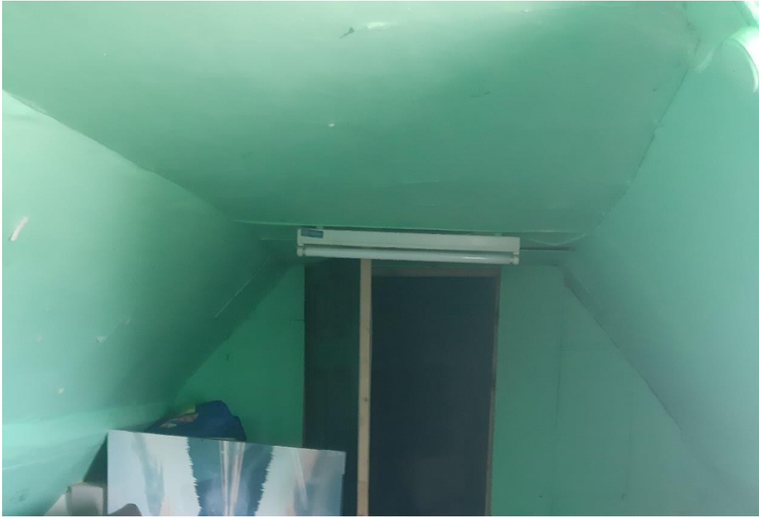
Photo 3: Southern attic space
