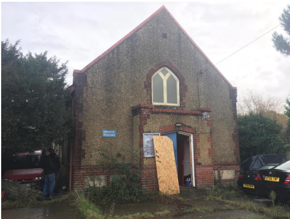
Figure 1: Methodist church, viewed from the west
