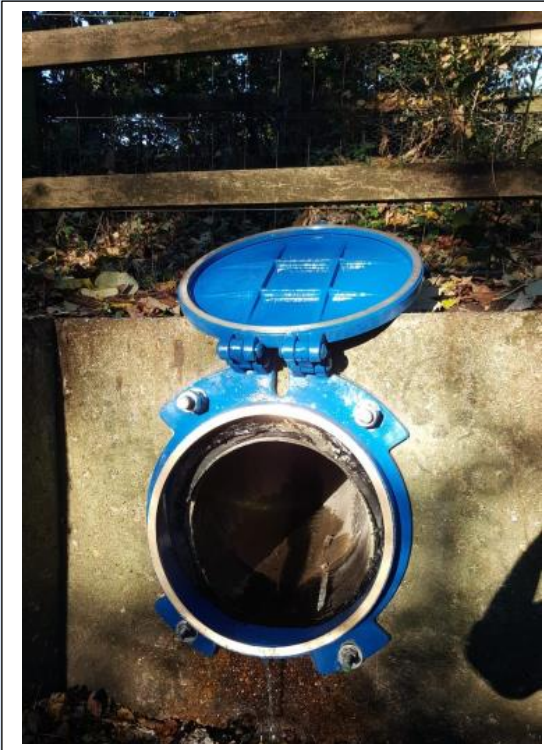
Image 1: Flap Valve fully open
