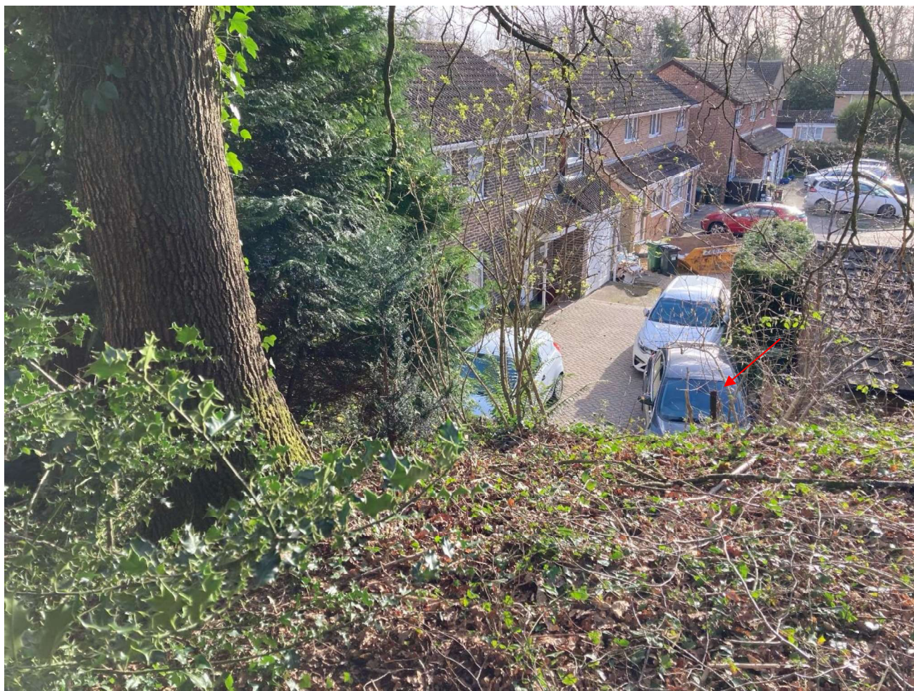
SAL3 'Peninsular' embankment top to east of no.58. Metal post identified by red arrow with garage behind and to the right / west of the post.
