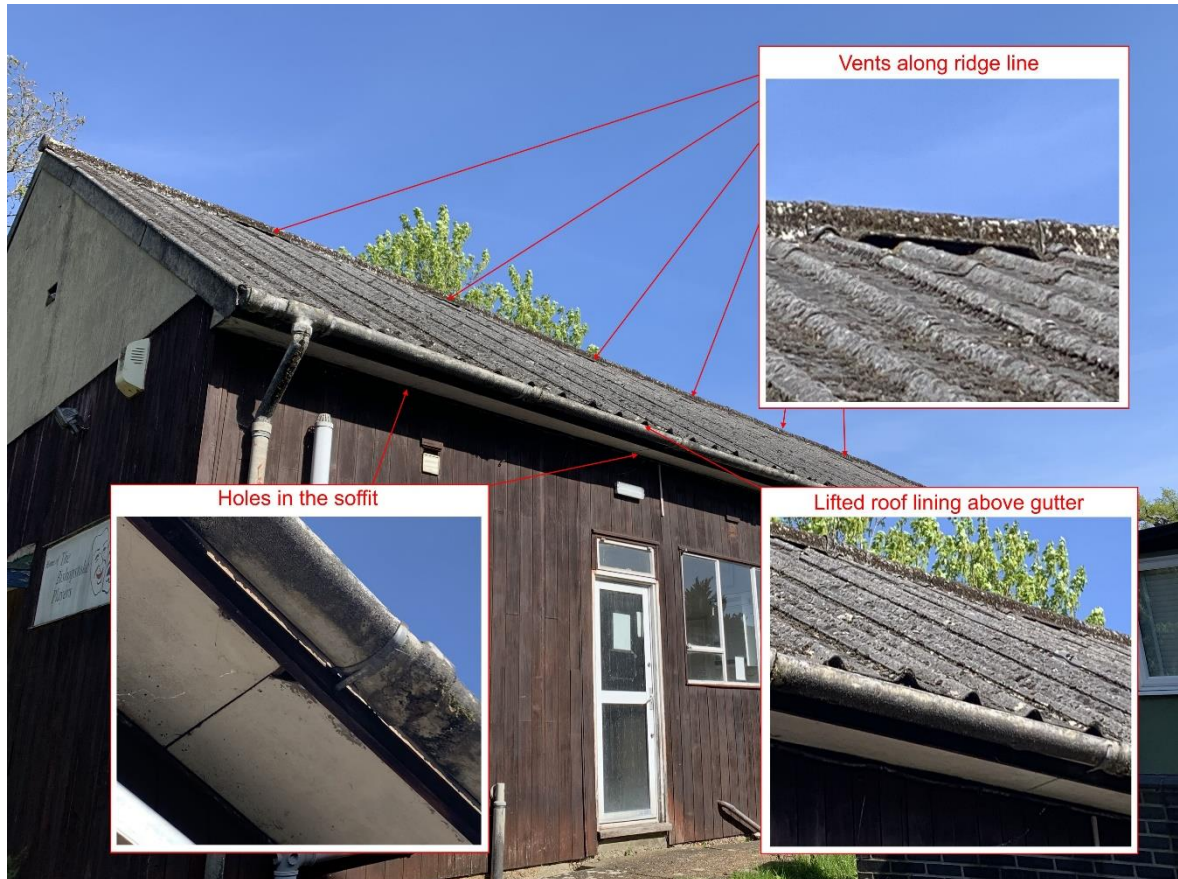
Image 4.3.1.3. Location of potential bat access points and potential external roost locations on the south elevation of the Memorial Hall.
