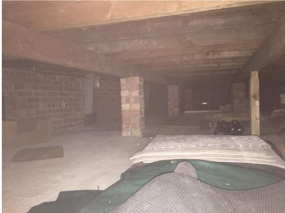
Photograph 9:- Below stage void and stage structure. Note portal leg and cleat fixing to LHS.
