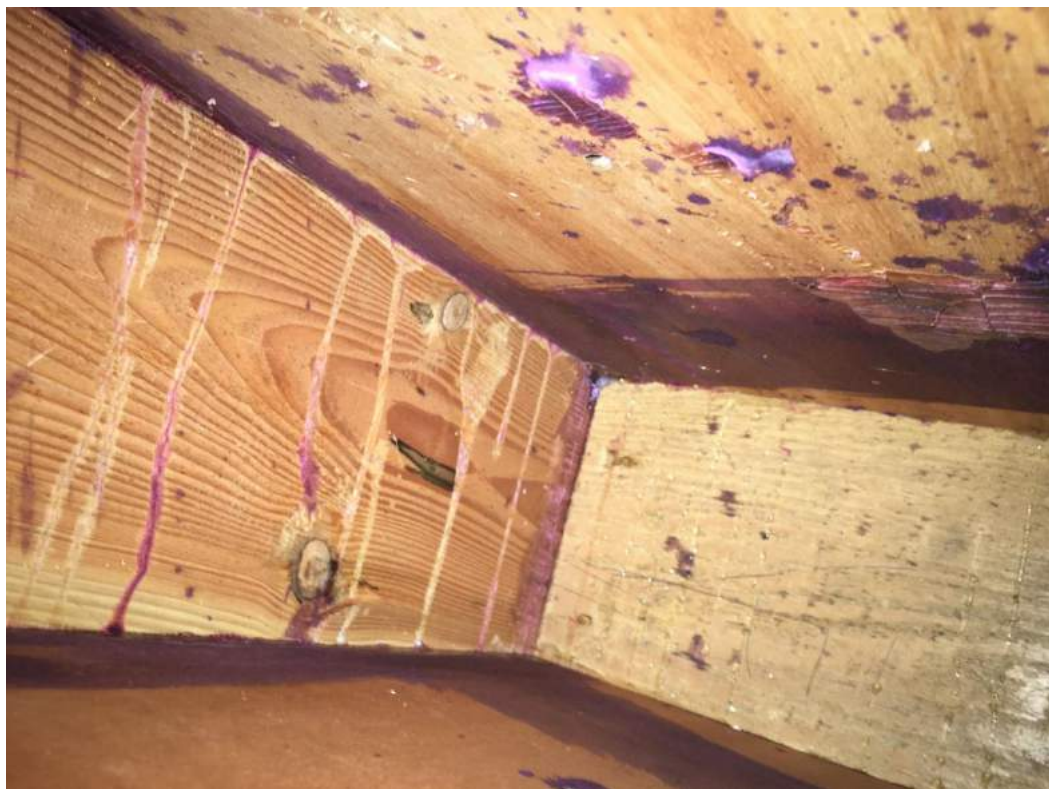
Photograph 14:- Internal view of portal construction
