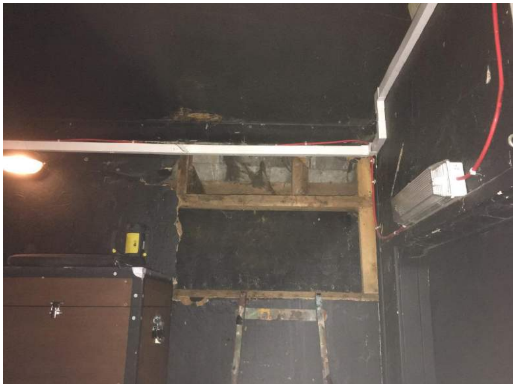
Photograph 16:- External wall construction at eaves level
