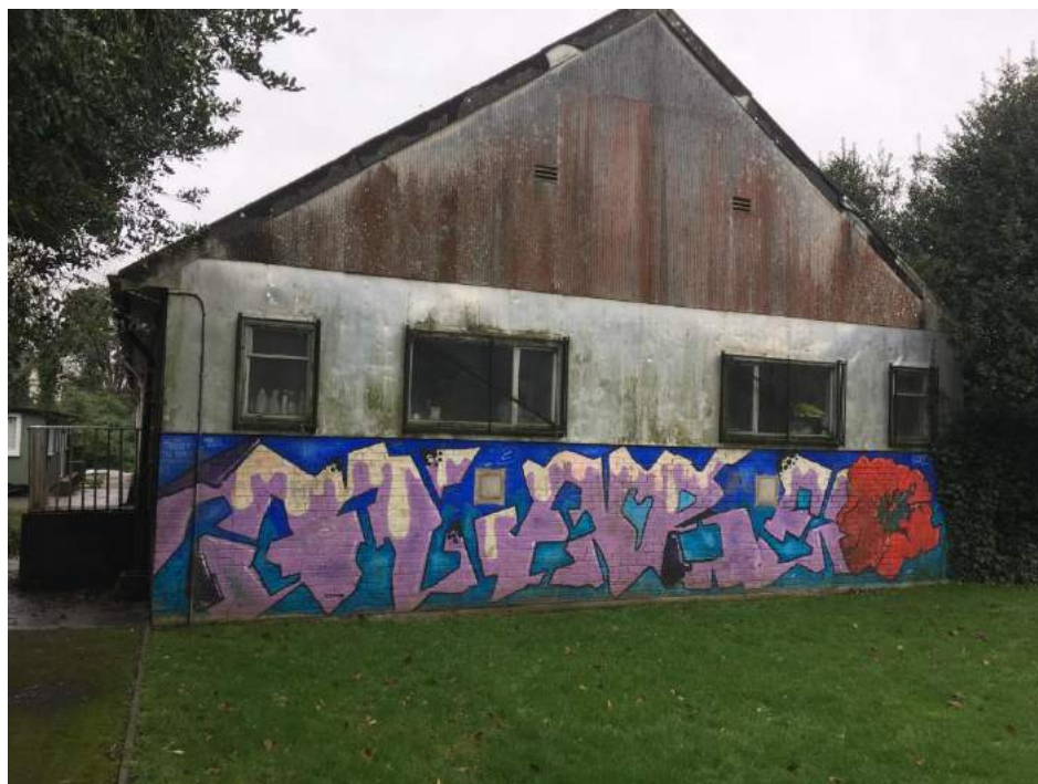
Photograph 2:- Rear - Northern Elevation
