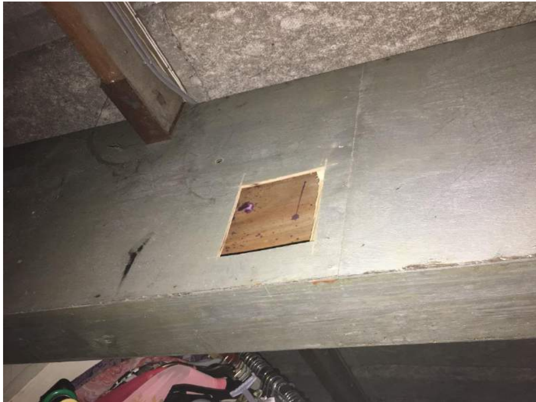
Photograph 13:- Extg hole cut in ply side wall of portal rafter
