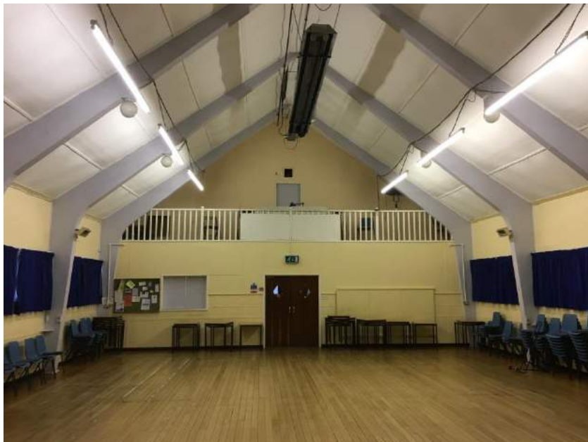
Photograph 6:- Hall viewed towards entrance
