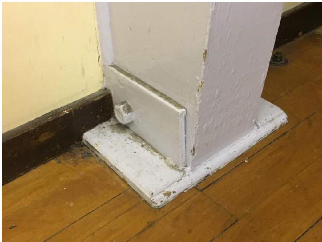
Photograph 8:- Typical cleat fixing at base of portal
