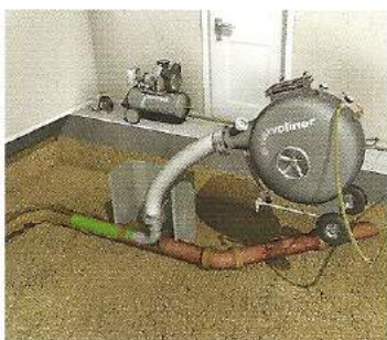
Inversion with a pressure drum
