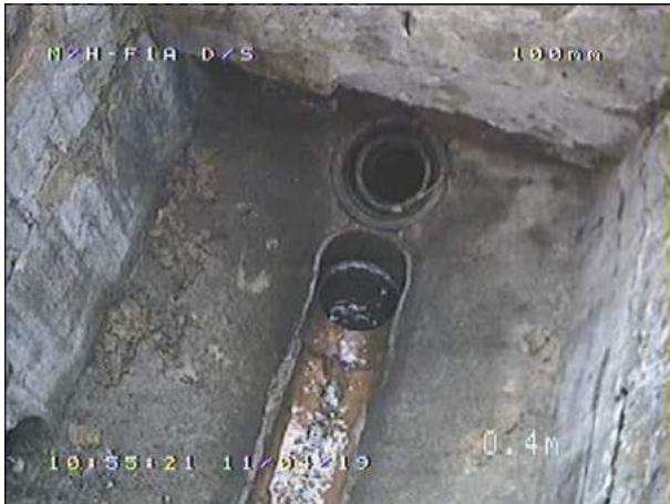
Photo: 11_11_77_A.JPG 0m, Start of survey
