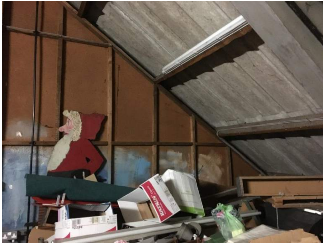
Photograph 11:- Internal wall to balcony and roof purlin / covering
