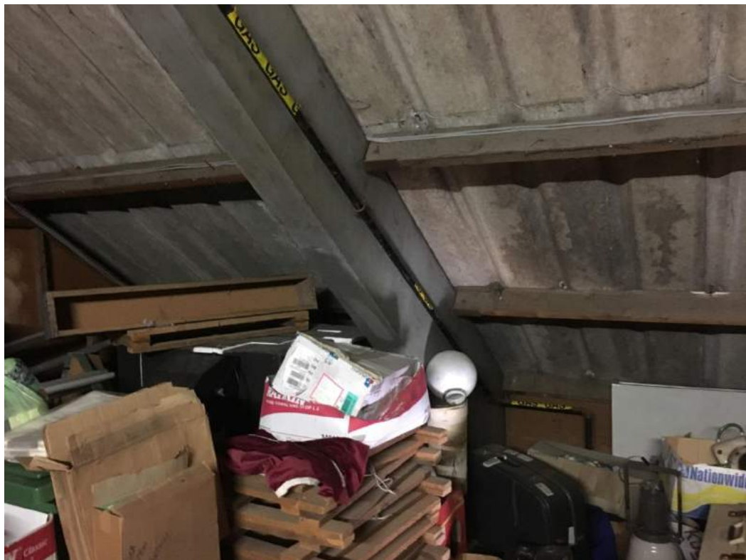
Photograph 12:- Typical purlin to portal rafter connection
