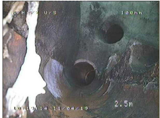
Photo: 3_3_32_A.JPG 2.5m, Manhole
