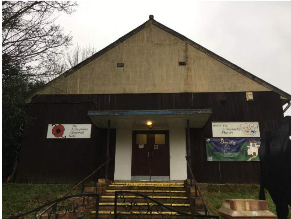
Photograph 1:- Front - Southern Elevation
