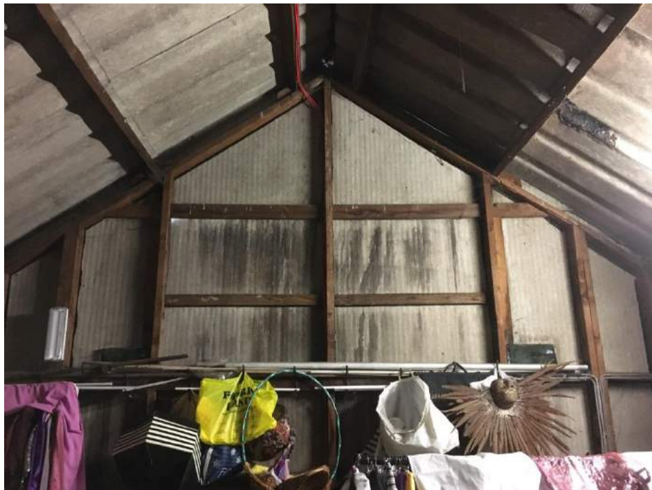
Photograph 10:- Front gable framing
