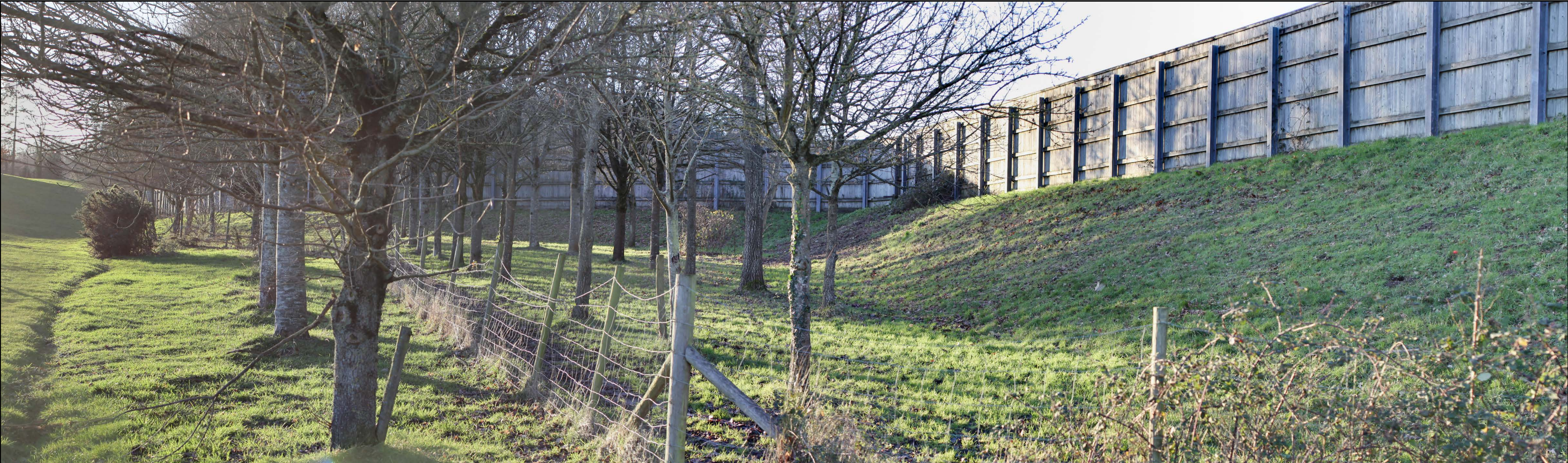
Viewpoint VP2 View from Public Right of Way (Ref: 241:509) along south-east site boundary looking west / north-west to boundary screen fence and earth mounding.
