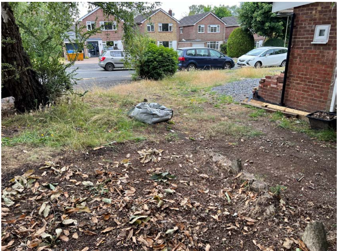
Photograph 4: Showing Tree 2 and the proximity to the newly constructed porch
