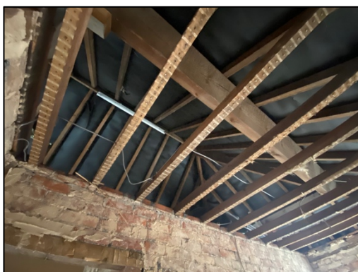
Figure 3 – open interior with exposed bitumen lining
