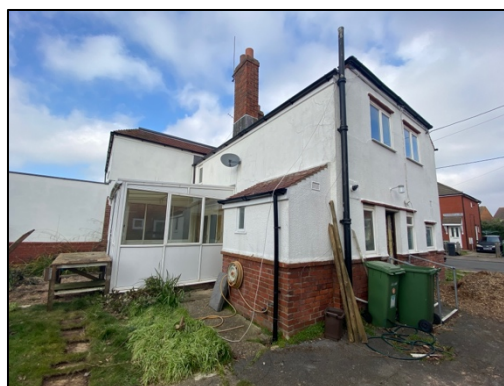
Figure 2 – rear conservatory and brick-built extension
