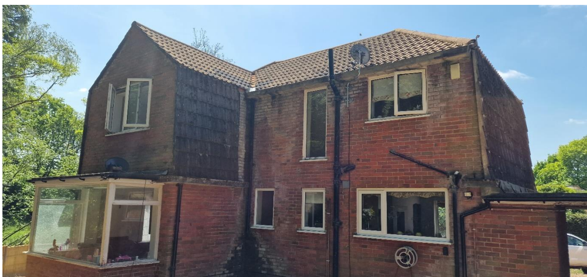
Picture 2: Showing the rear elevation of the building.
