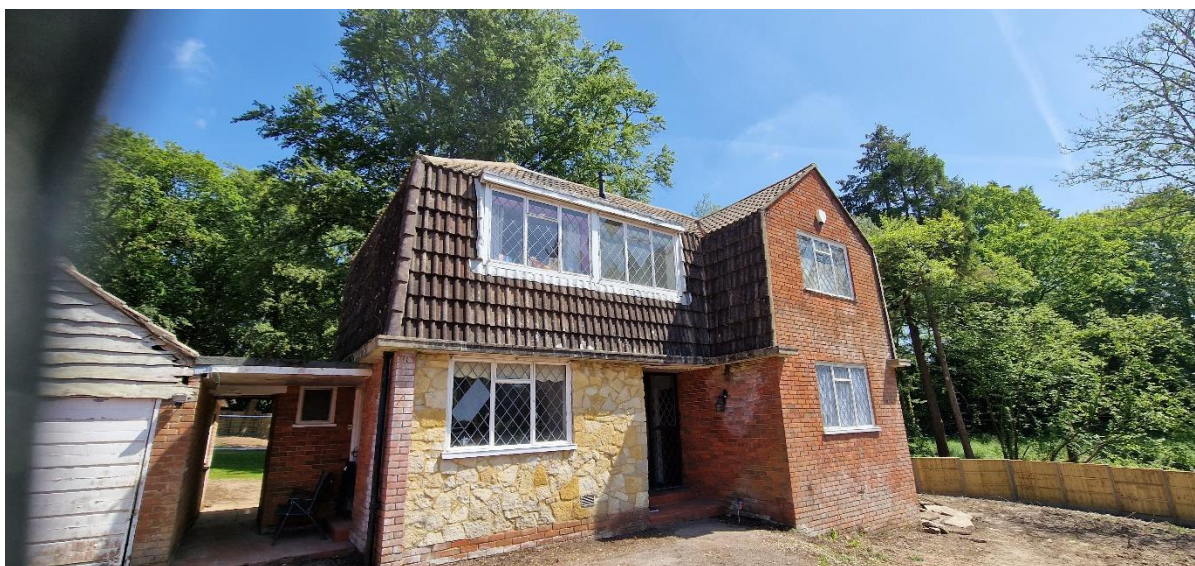
Picture 1: Looking at the front elevation of the building.
