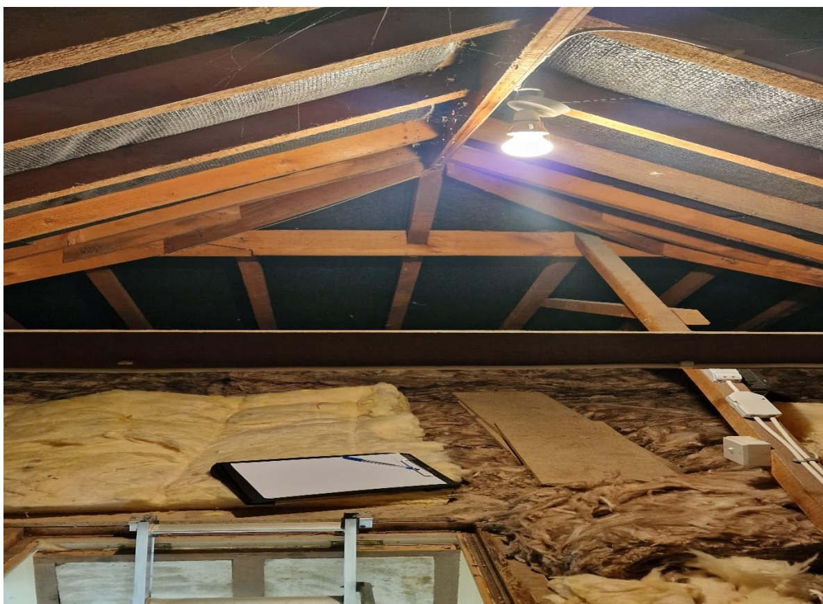
Picture 4: Showing the roof void.
