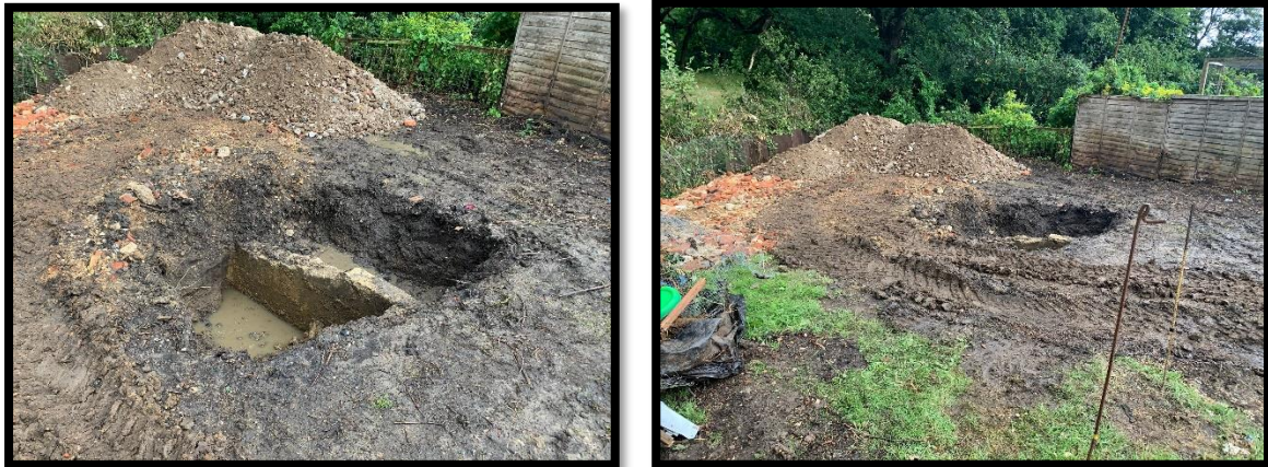
Plate 1: Defunct cesspit location and excavated evidence.
