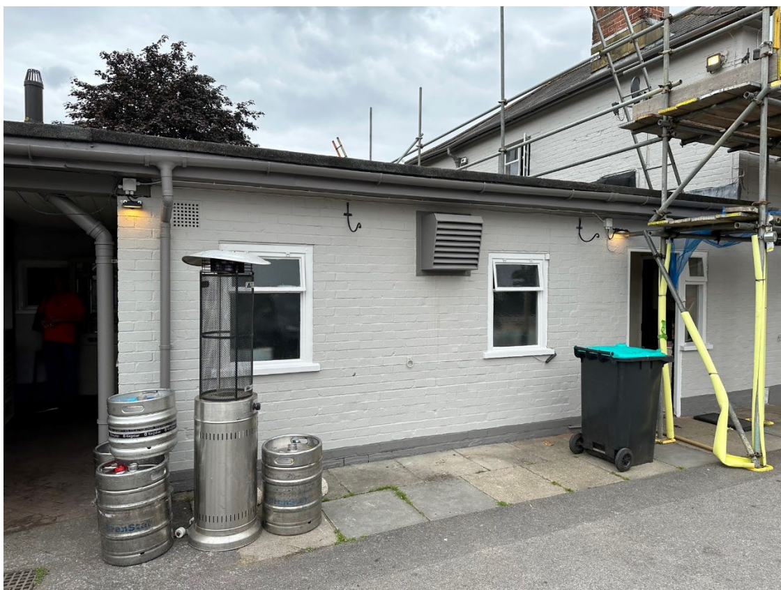
Photo showing the rear kitchen area, and extraction unit to be replaced
