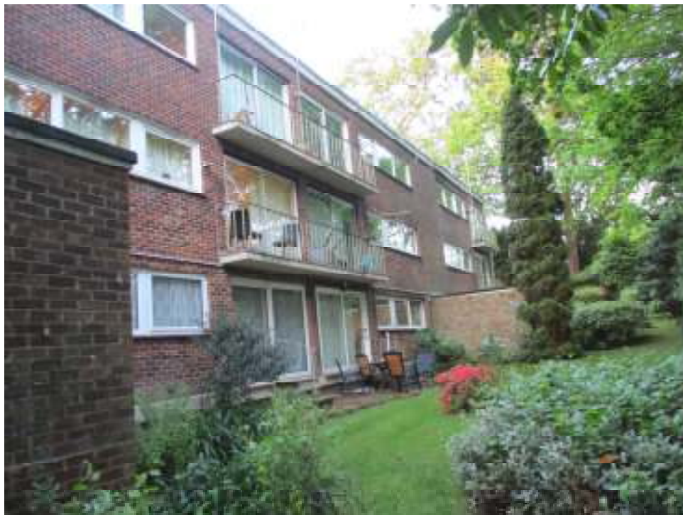
A view of the rear of the building
