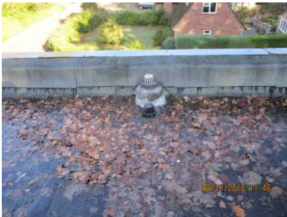
A view of the leaf litter around an outfall
