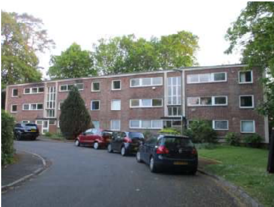
View of the front of the building
