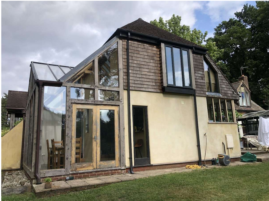
Photo 7: West elevation of north wing
