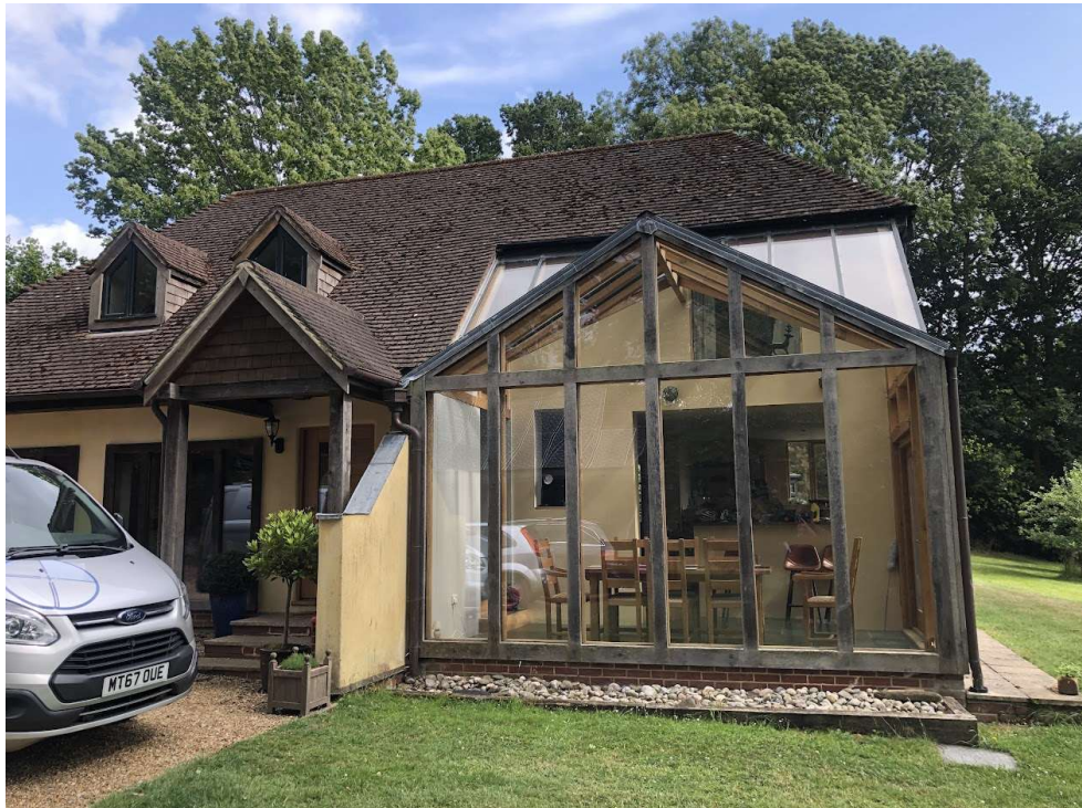
Photo 1: Front north elevation.
