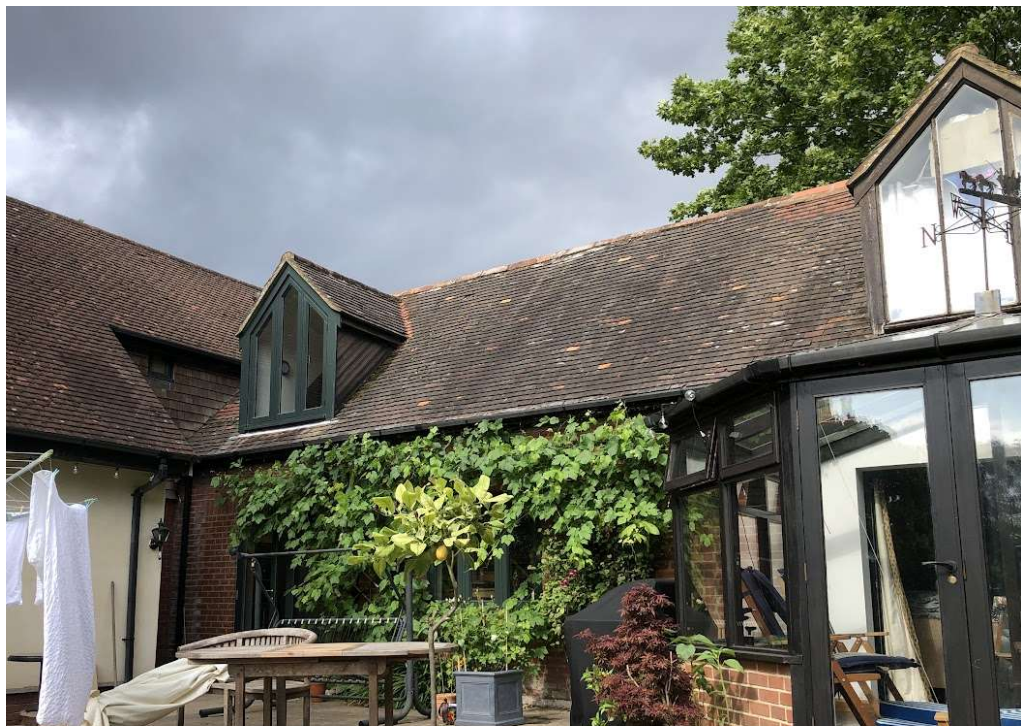
Photo 6: West elevation of south wing
