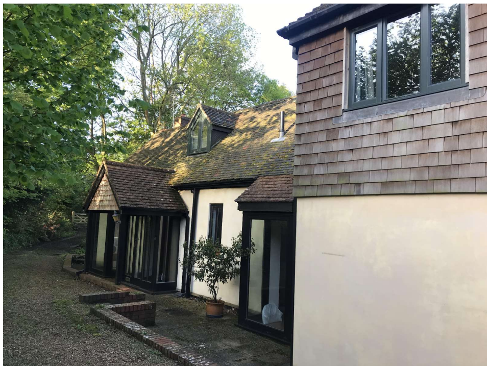
Photo 4: East elevation of south wing
