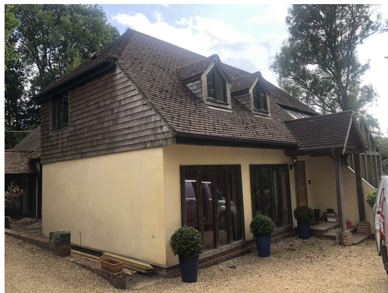
Photo 2: North and part east elevation
