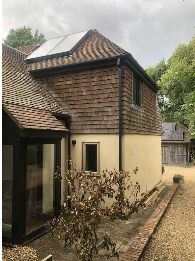
Photo 3: East elevation of north wing
