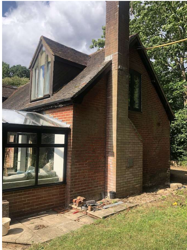
Photo 5: South elevation of south wing gable end
