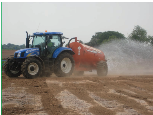
Figure 4.29 Dust suppression (courtesy Galliford Try plc)
