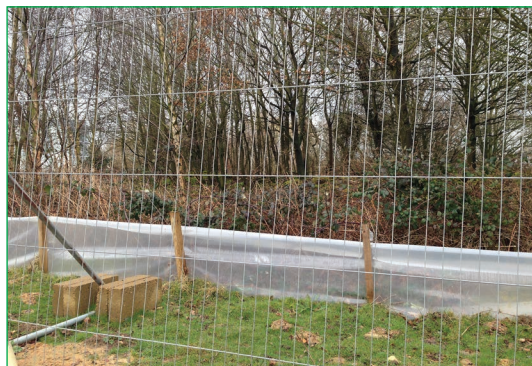
Figure 4.14 Great crested newt fencing (courtesy Brookfield Multiplex)
