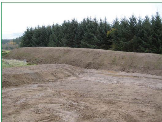
Figure 4.45 Landscaped stockpile of spoil (courtesy Galliford Try plc)
