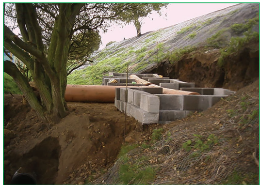
Figure 4.9 Badger sett construction (courtesy BAM Nuttall)
