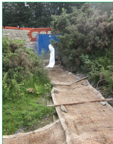
Figure 4.58 Dirt box, silt sock and sedimats
