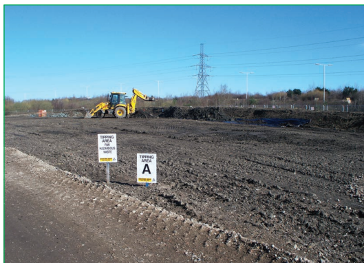
Figure 4.27 Land remediation (courtesy Parsons Brinckerhoff)
