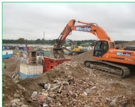
Figure 4.42 On site crusher (courtesy Skanska)
