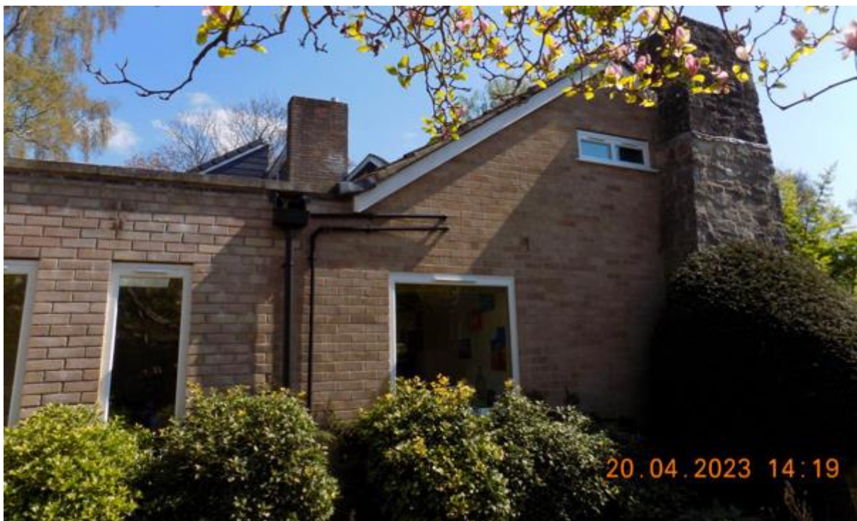
Image 4 – West facing elevation of the property
