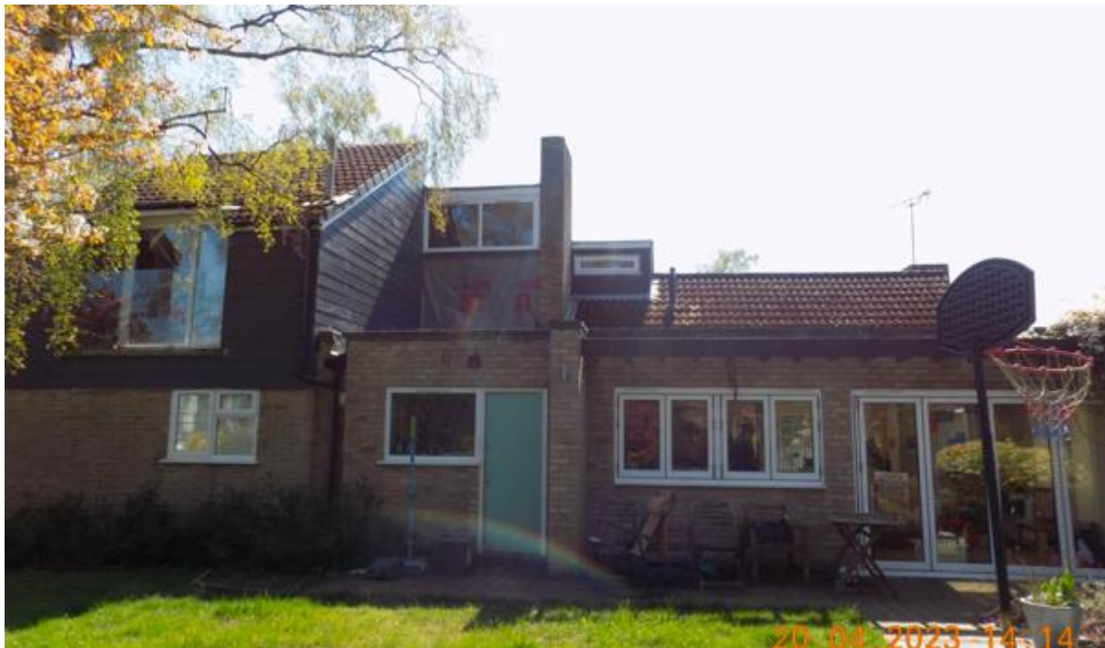
Image 3 – North facing elevation of the property
