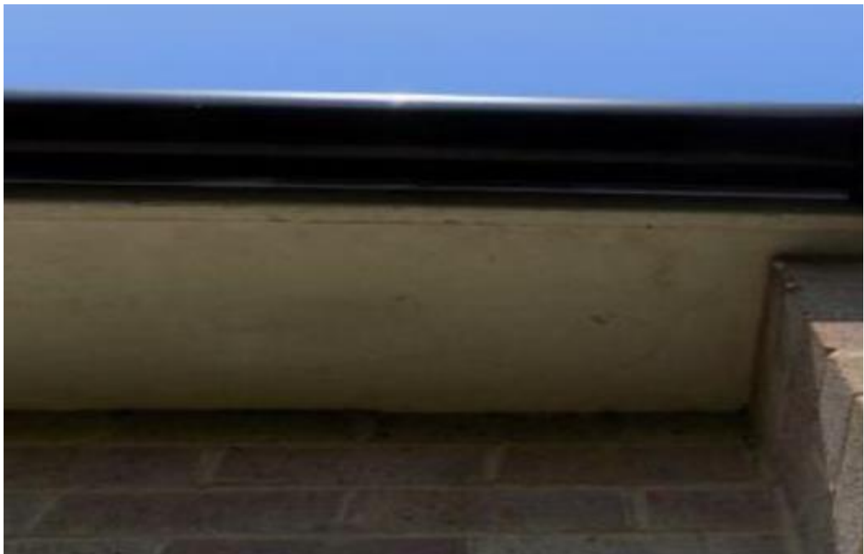
Image 6 – Close view of the main eaves coverings which have demonstrated a fair level of condition throughout
