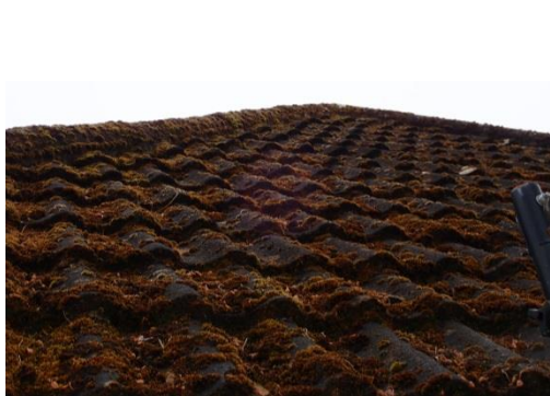
Tightly-fitting roof tiles
