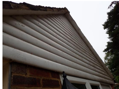
Tightly-fitting cladding on rear gable
