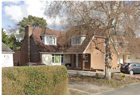
Fig.9 – 174 Hiltingbury Road – appears to have had the roof space remodelled for first floor accommodation. Similarities with no. 150 (may have started with similar design)
