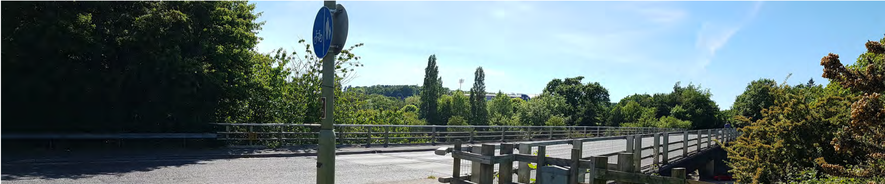
KEY REPRESENTATIVE VIEWPOINT 8 - View from B3035 Botley Road looking south at M27 bridge and Public Right of Way 10.
