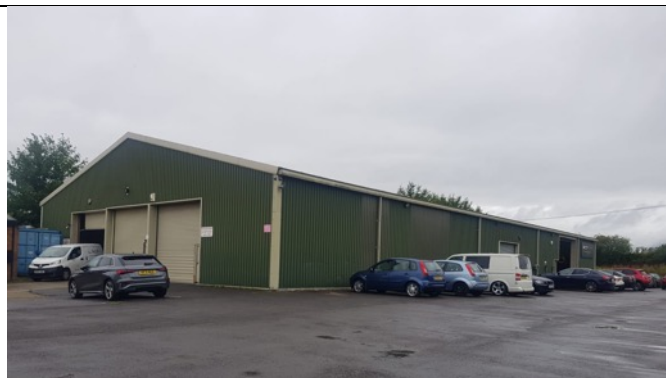
Photograph 1. B1, with hardstanding tarmac in foreground.
