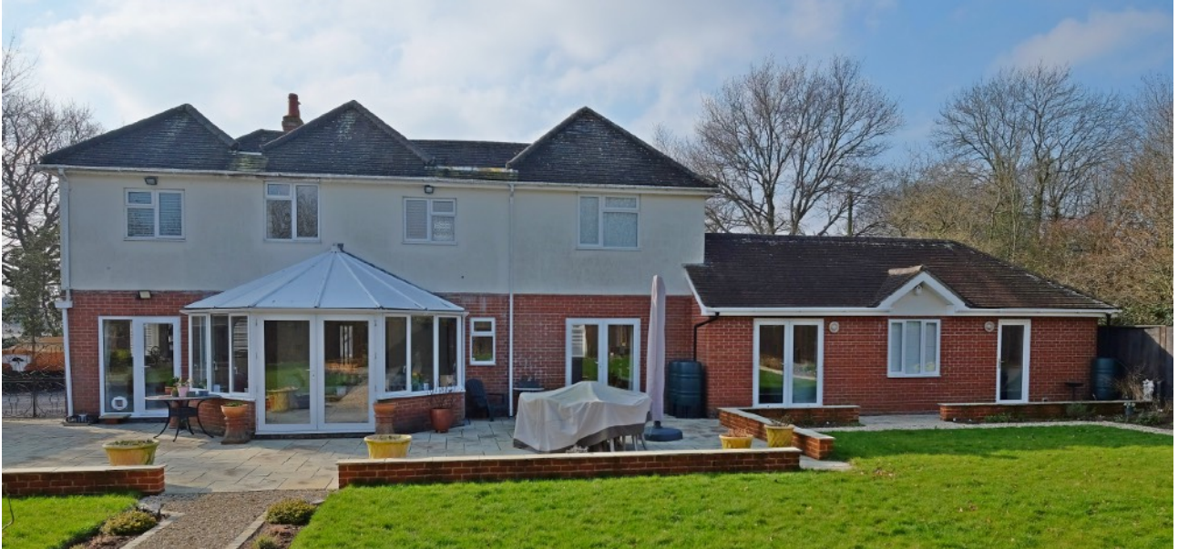
Figure 2 Existing Rear North Elevation
