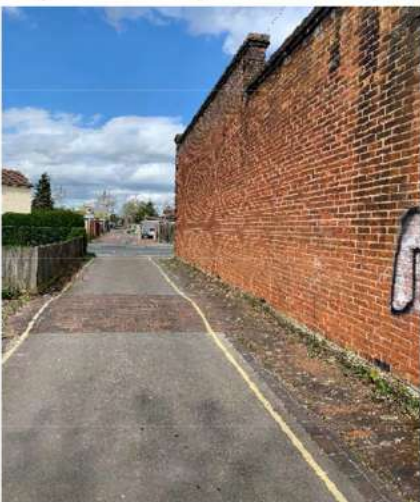
Image 5 – West Service Road looking north
