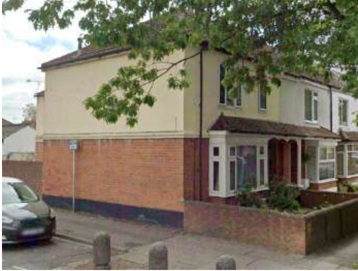
Red brick to ground floor with contrasting coloured render to first floor
