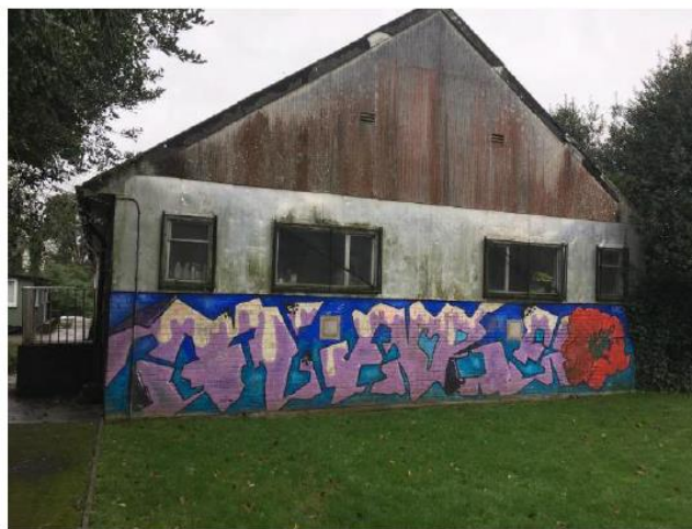
Photograph 2 - Rear Northern Elevation
