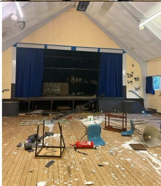
Photograph 6 Hall view towards stage
