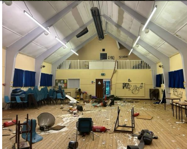
Photograph 5 - Hall view towards entrance
