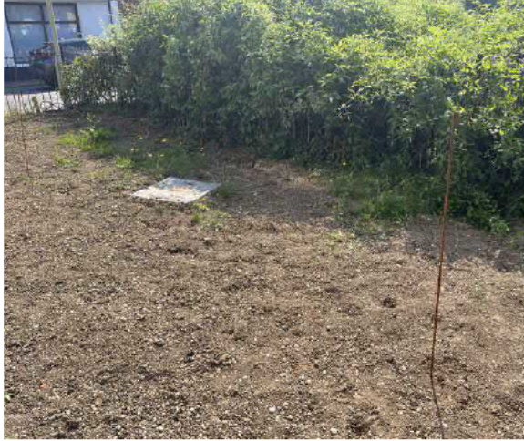
Photograph 1 Overview of VP101 prior to excavation
