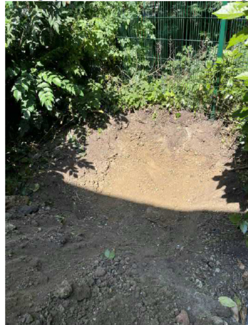
Photograph 4 VP102 Excavated to 450mm bgl
