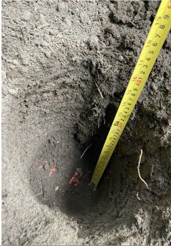
Photograph 9 HP303 Validation Pit
