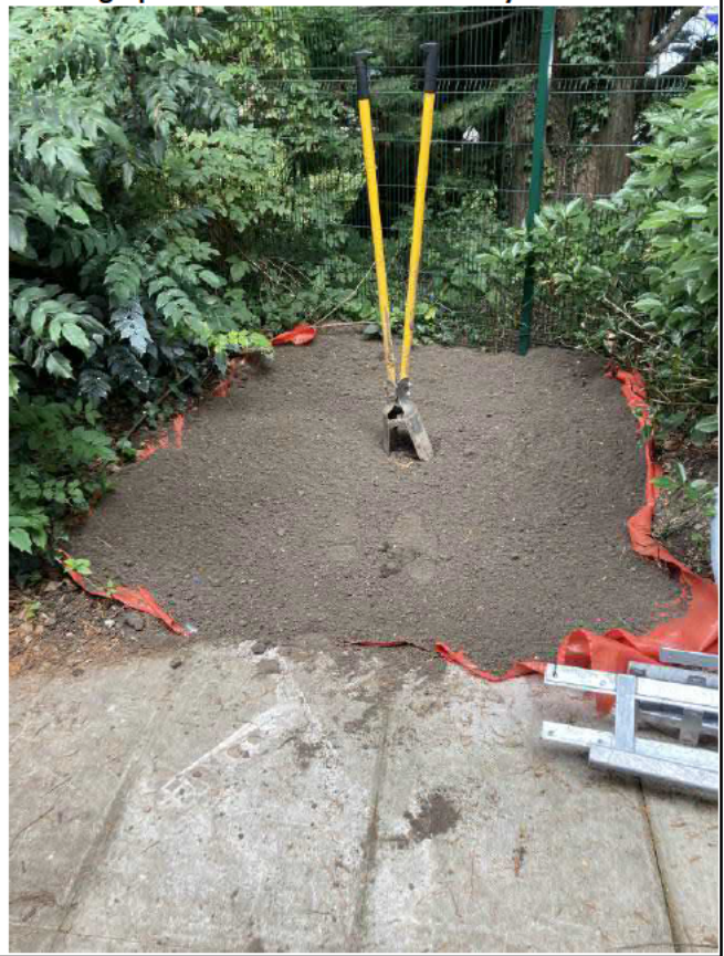
Photograph 6 VP102 with clean cover system installed
