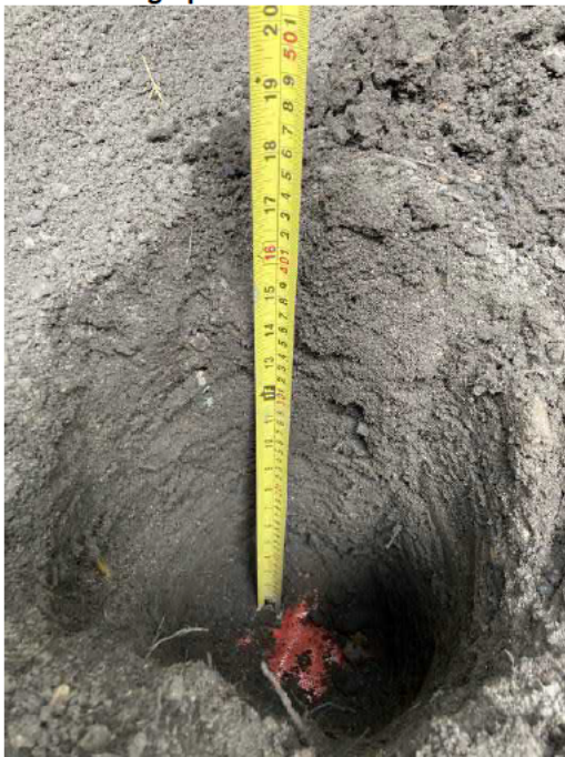
Photograph 7 HP302 Validation Pit
