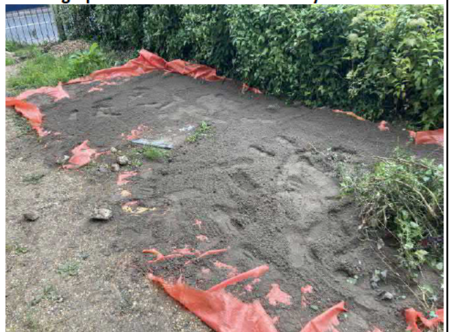
Photograph 8 VP101 with clean cover system installed
