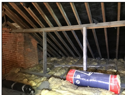
Figure 4 – internal view of the roof void, facing south-west.
