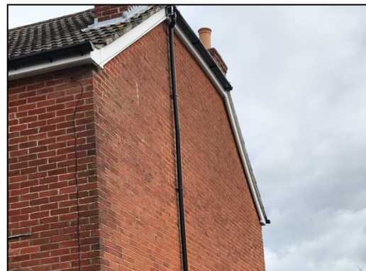
Figure 2 – south-eastern elevation of the house
