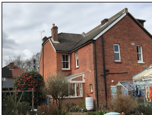
Figure 3 – north-eastern elevation, also showing the conservatory at side elevation.
