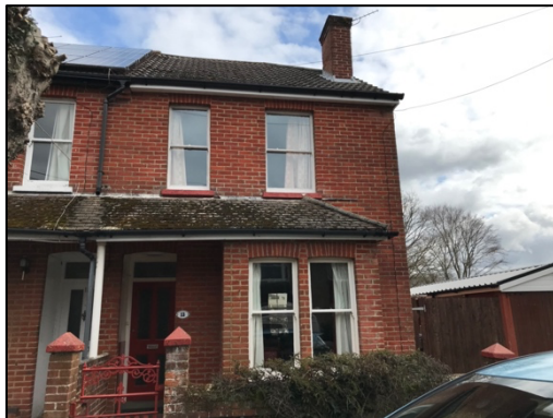
Figure 1 – south-western elevation of house
