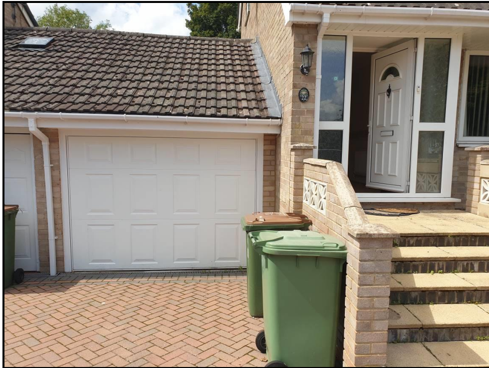
Existing Attached Garage
