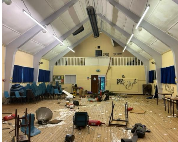
Photograph 5 - Hall view towards entrance
