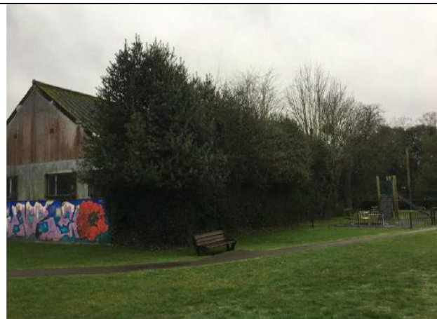
Photograph 3 - Mature Trees close to western side of building
