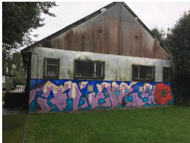
Photograph 2 - Rear Northern Elevation
