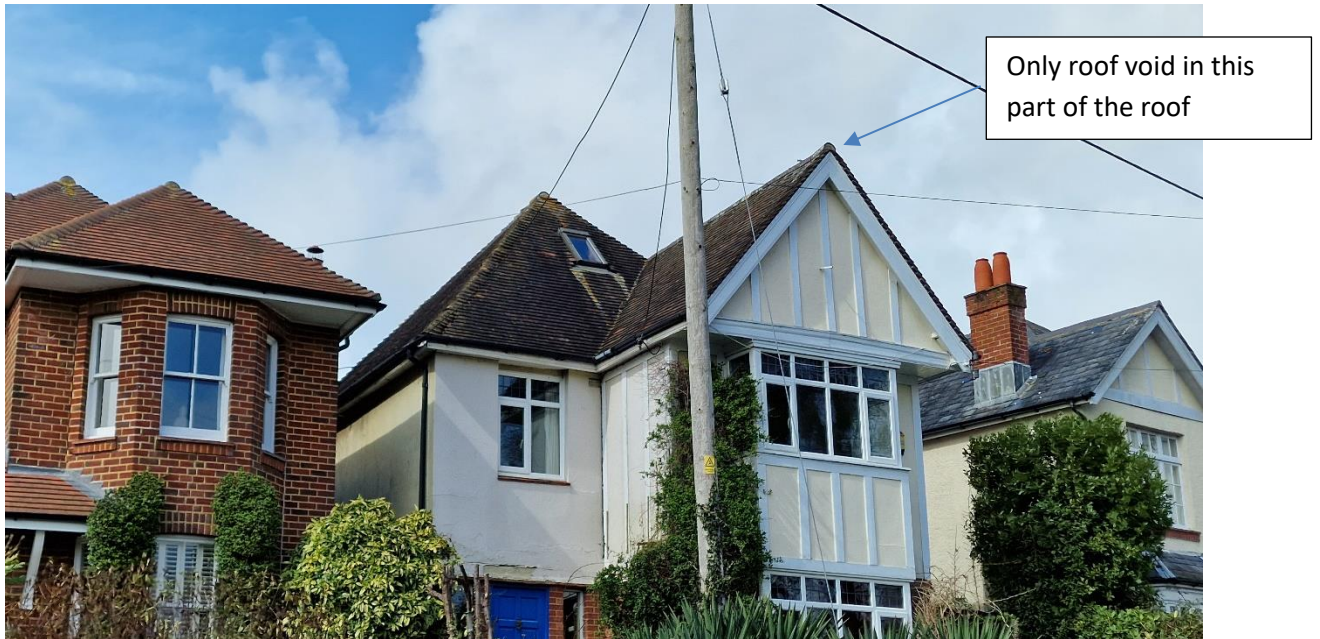
Picture 1: Looking at the front elevation.
