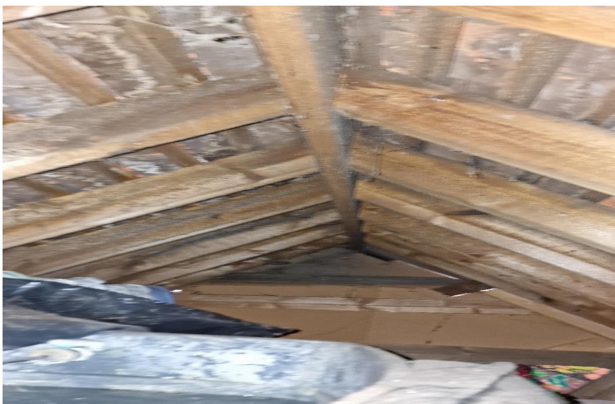
Picture 4: Showing the roof structure in the accessible roof void.
