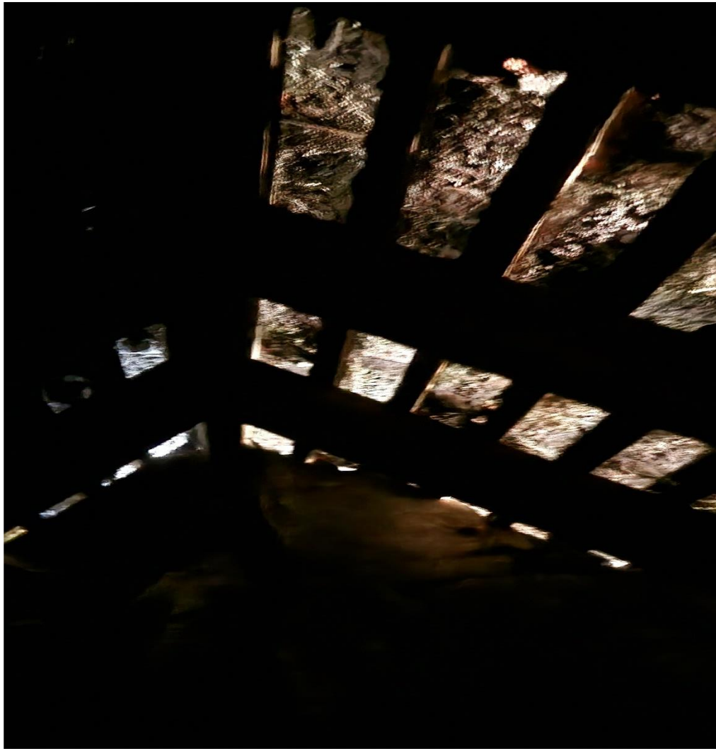
Picture 5: Showing the small roof void with the light coming in from outside.
