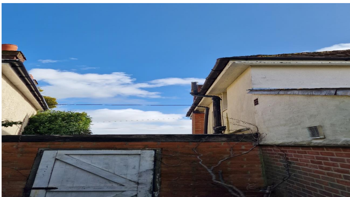
Picture 3: Showing the tight-fitting eaves.
