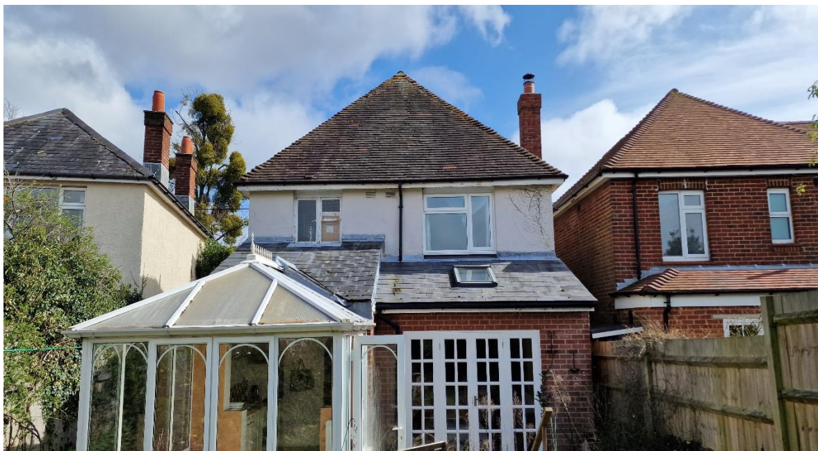
Picture 2: Showing the rear elevation of the building.
