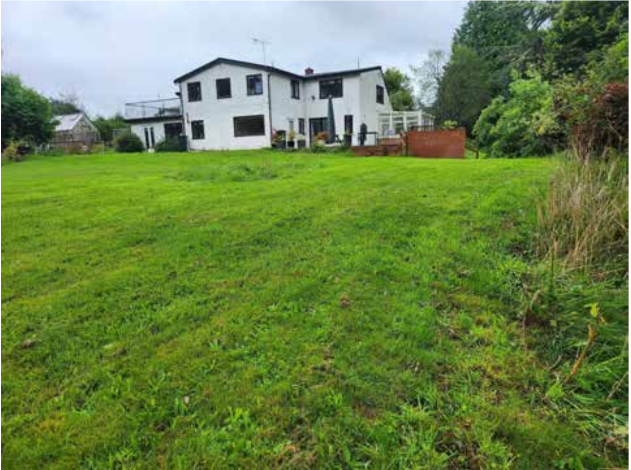
Plate 14 View of the rear of the residential property
