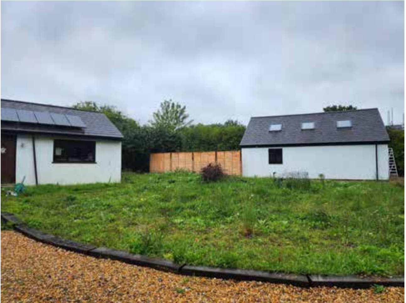
Plate 4 View of the two single storey outbuildings/garages
