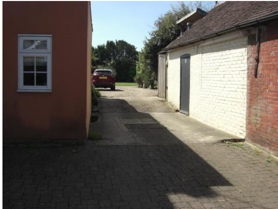
Existing side access leading to rear driveway
