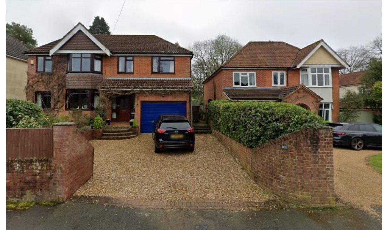
No.s 99 & 101 two storey flat façade side extensions to original dwellings, 99 with central flat roof
