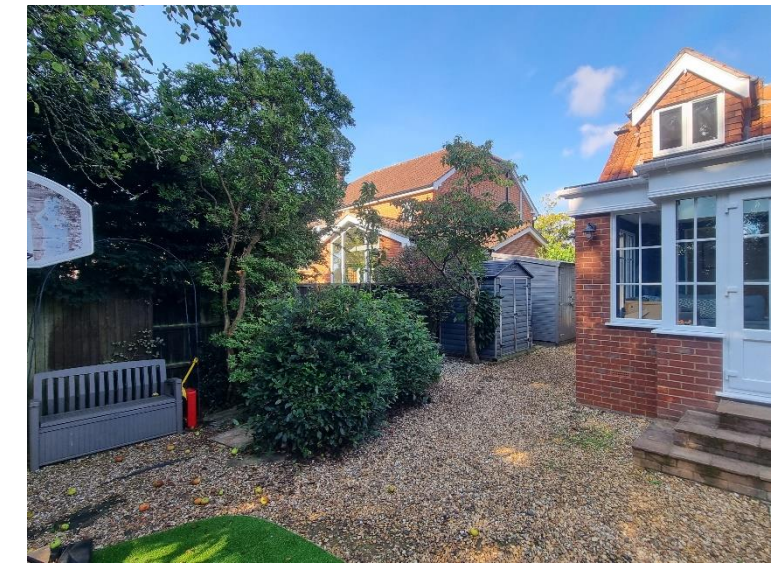
Obstructed views towards No.95, 95 rear extension.
