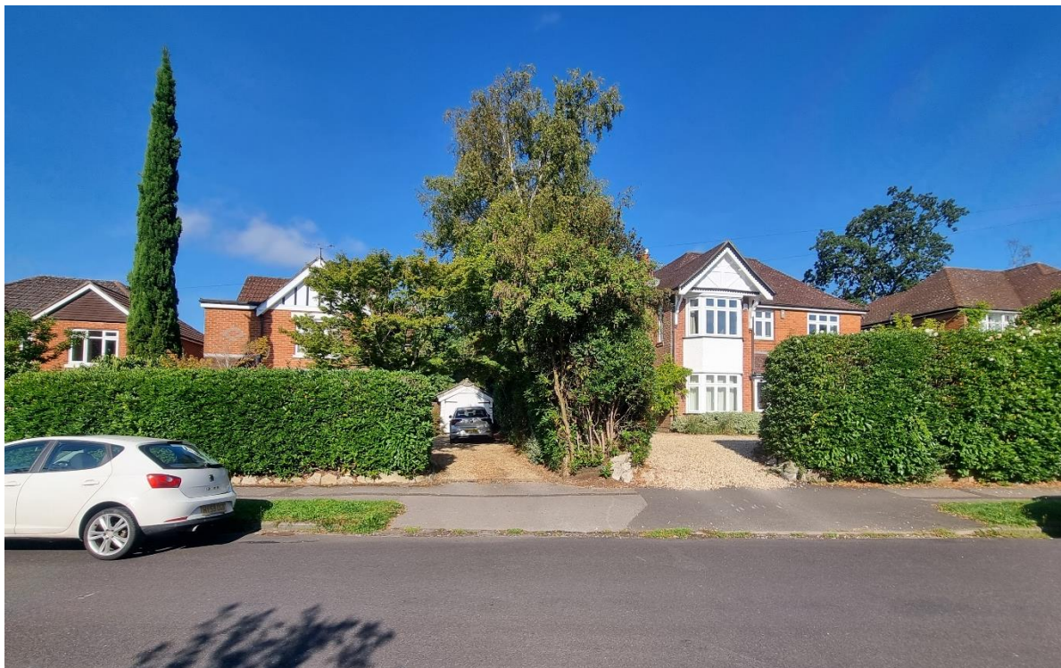
Directly opposite 97 Kingsway, two storey flat façade side extensions with flat and pitched roofs
