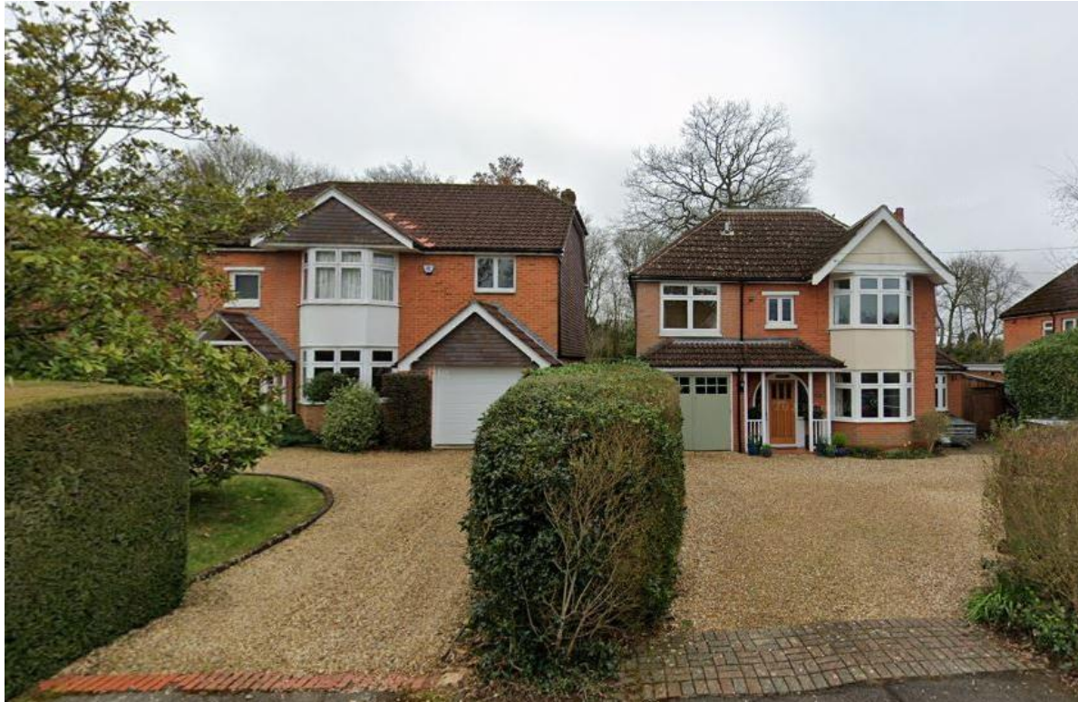
No.s 93 & 95 two storey flat façade side extensions to original dwellings, 93 with central flat roof
