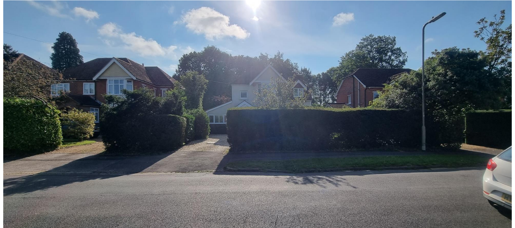
Kingsway street scene and boundary treatment, facade facing North West.
