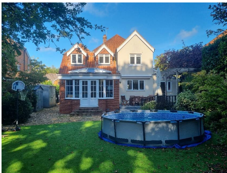
Scale/ style of rear roof out of keeping with neighbours
