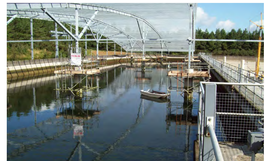
Above: Roof construction in 2012 (source: structa.co.uk)
