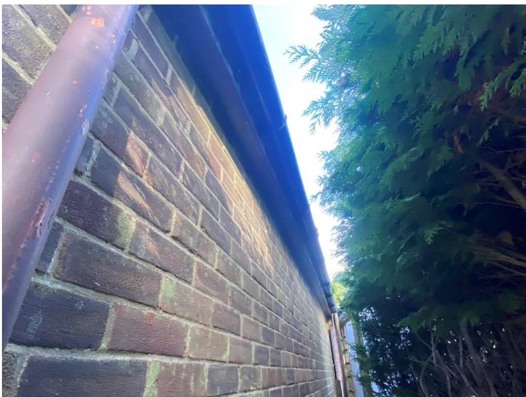
Figure 4. East face of garage looking north.
