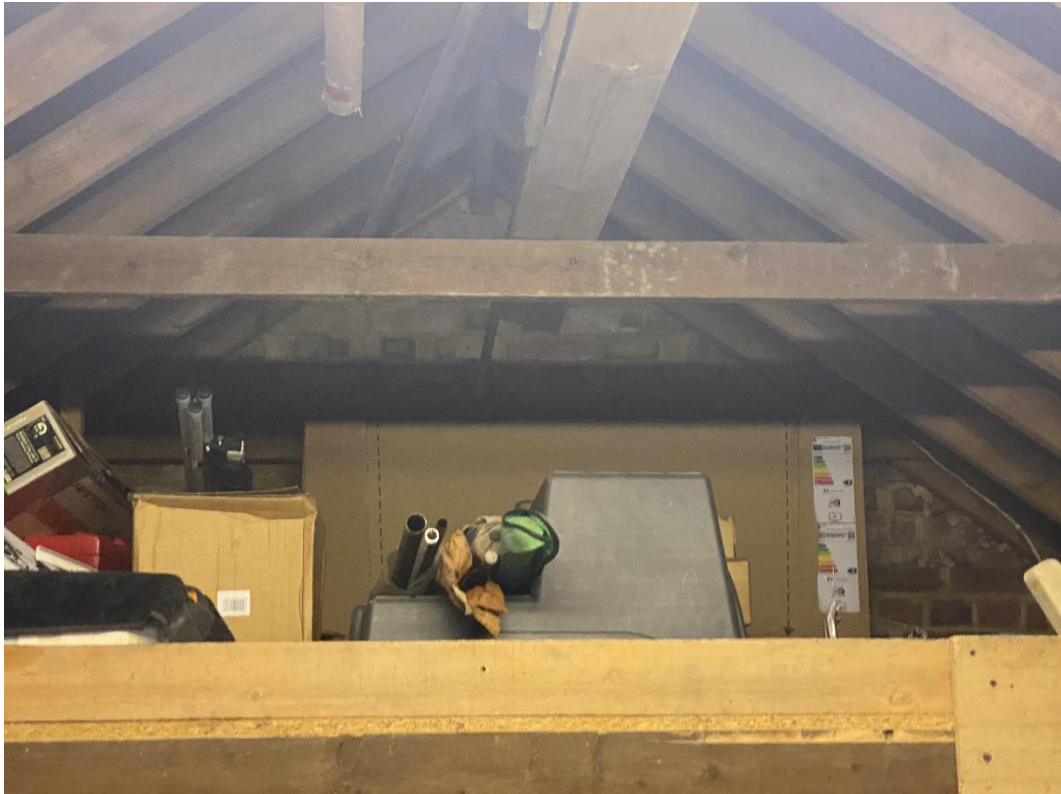
Figure 4. Inside of roof space looking south
