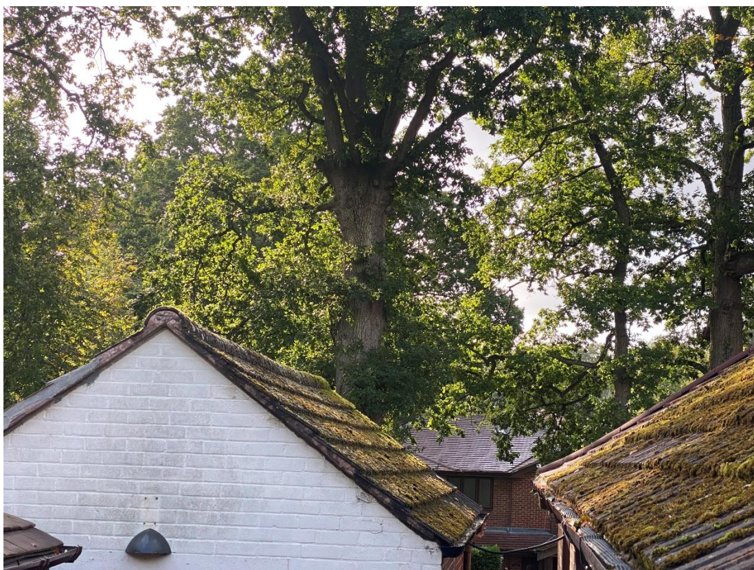
Figure 2. Western and northern elevations looking south.
