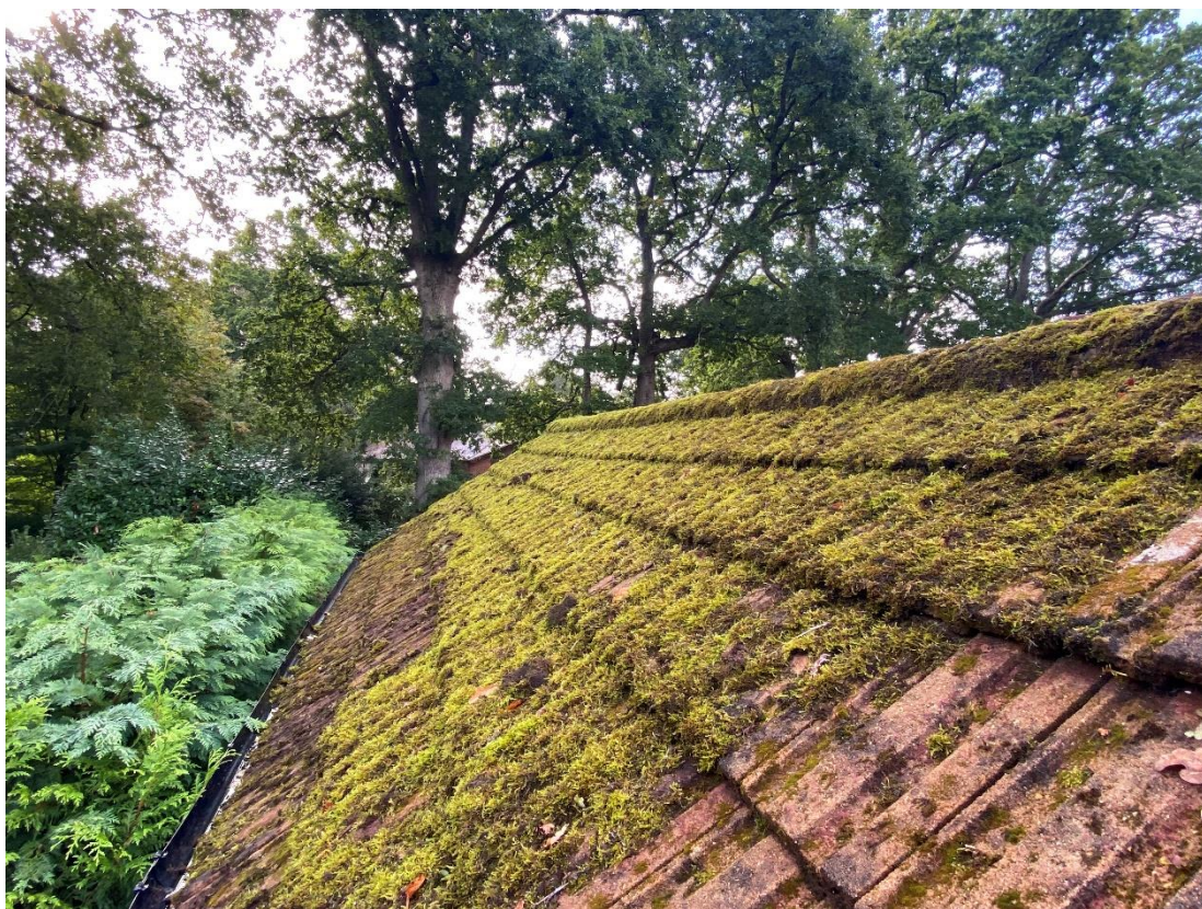
Figure 3. East face of roof looking south.
