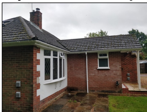
Figure 3 – southern gable end porch extension
