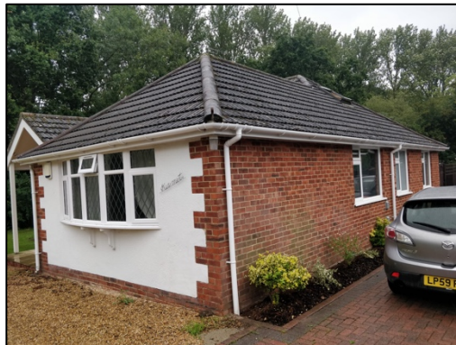
Figure 1 – south-eastern corner of the bungalow
