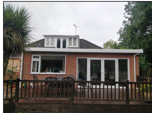
Figure 2 – northern elevations of the bungalow
