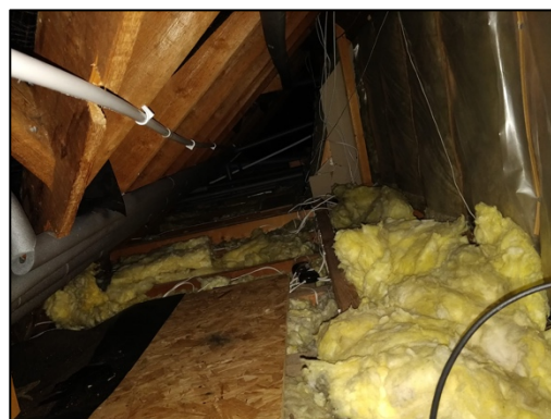
Figure 6 – roof void extending along the side eaves.
