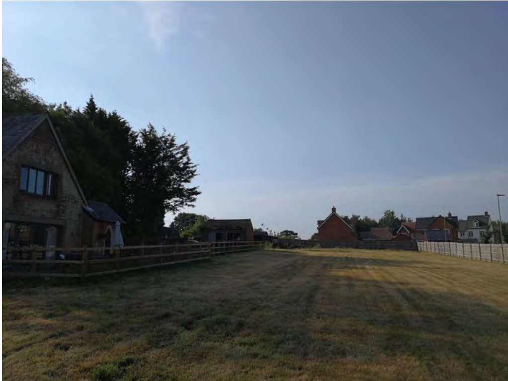
Figure 6. A view of the rear of existing Oakfields dwelling, with a small patio area located to rear adjacent to the amenity grassland (Ecosupport 2020).
